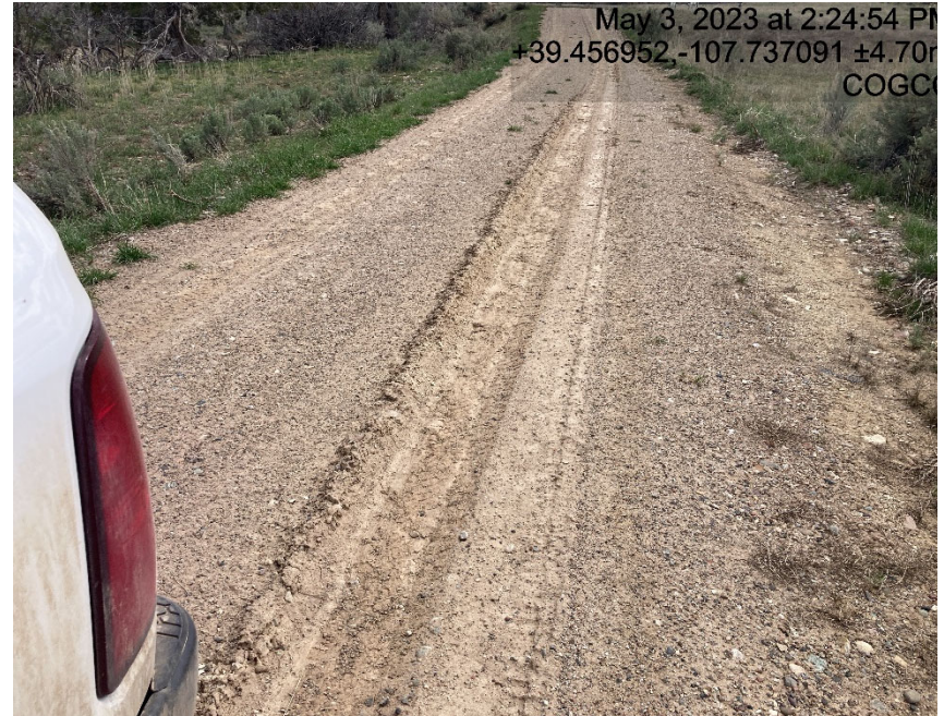
Lack of stabilization/compaction
