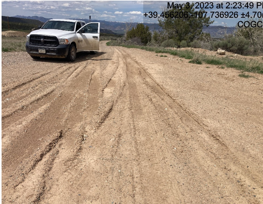
Lack of stabilization/compaction
