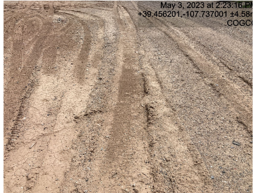
Lack of stabilization/compaction
