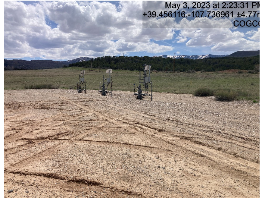
Location and Lack of stabilization/compaction
