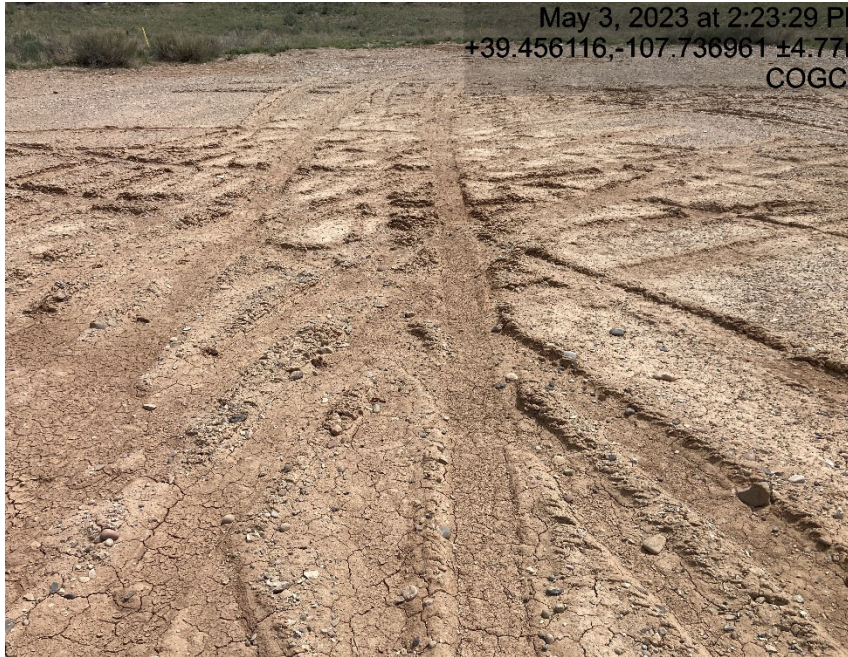
Lack of stabilization/compaction
