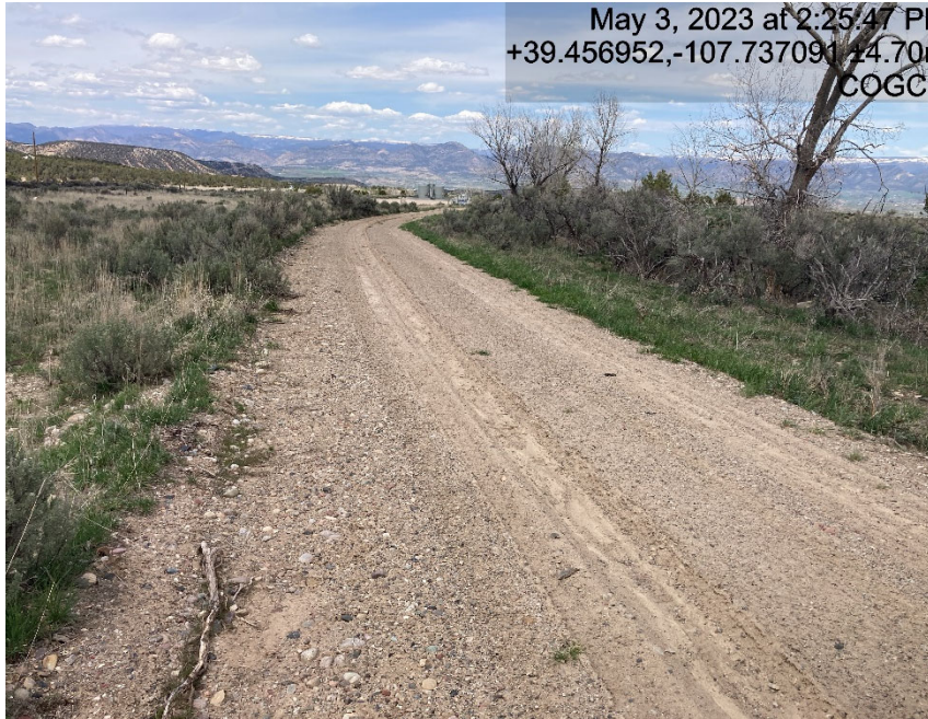
Lack of stabilization/compaction
