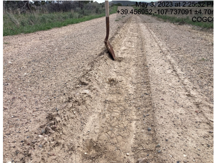
Lack of stabilization/compaction
