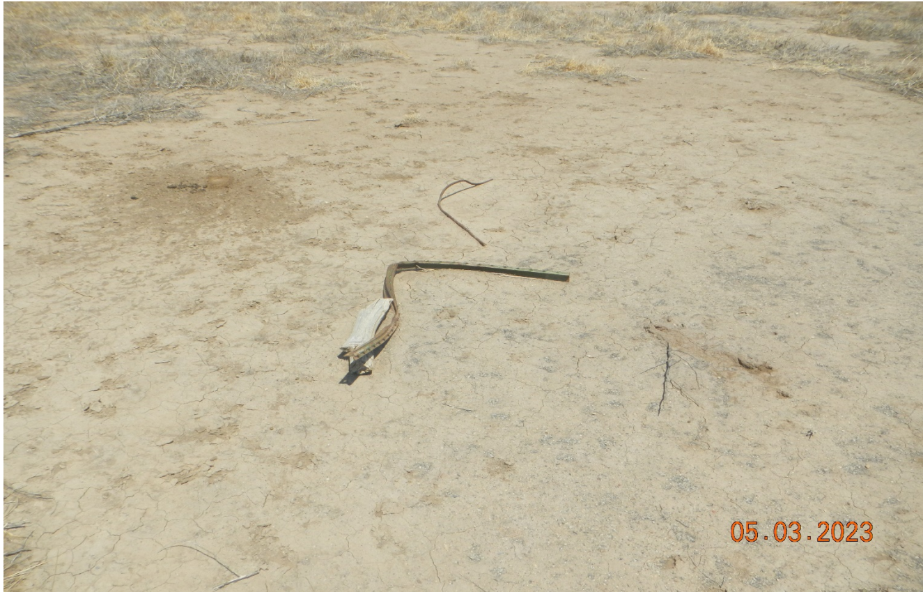
Photo 4. There is metal t-post and wire debris that needs to be removed.
