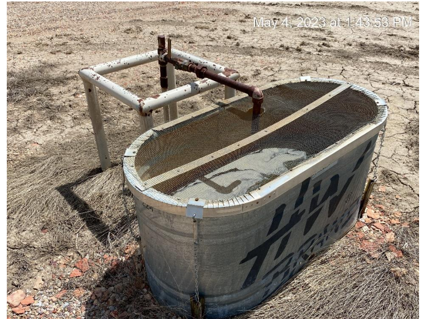
Liquid unloading tank. No secondary containment.
