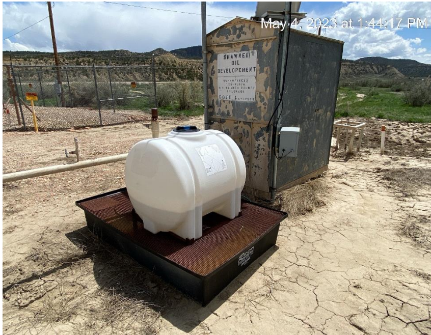
Chemical tank and gas meter run
