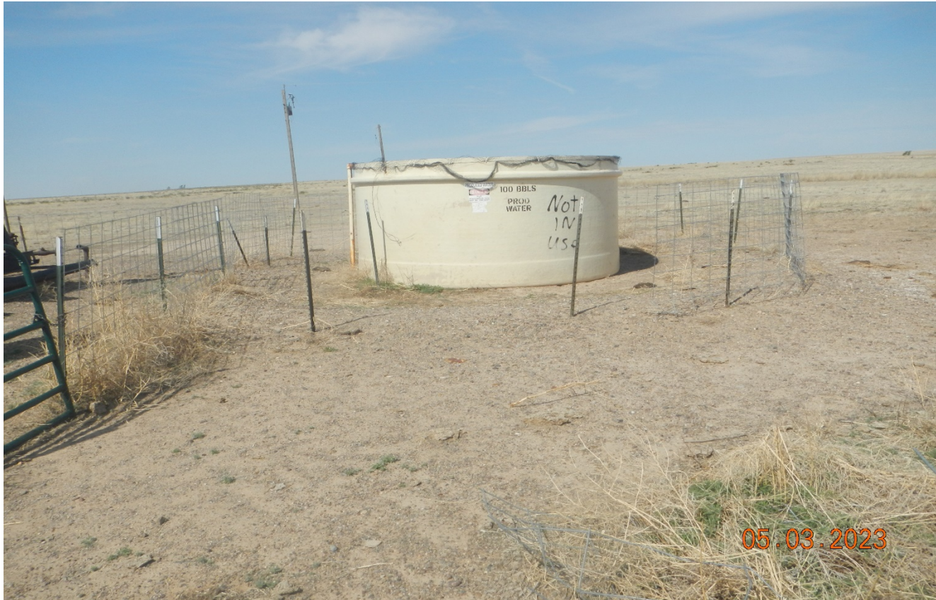
Photo 4. Facing toward the open top tank which still does not have secondary containment. The fence around the tank has fallen over in disrepair.
