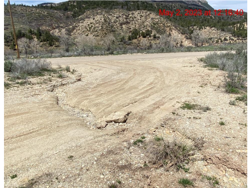
Rill Erosion Across Access Road/Insufficient Vehicle Tracking BMPs – Photo #02798
