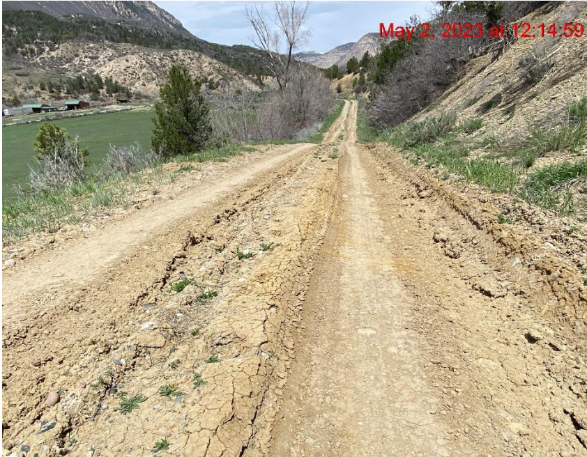
Access Road Lacks Stabilization – Photo #02797
