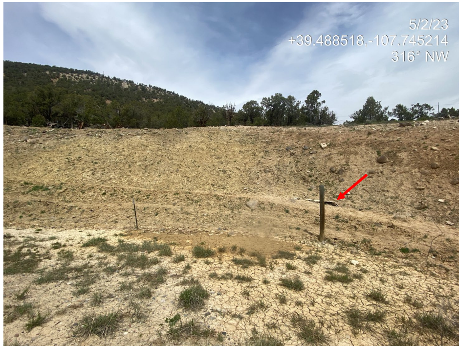
Photo 5. Photos show slopes to the northwest of the location lack stabilization. Photo also shows dead livestock (left).
