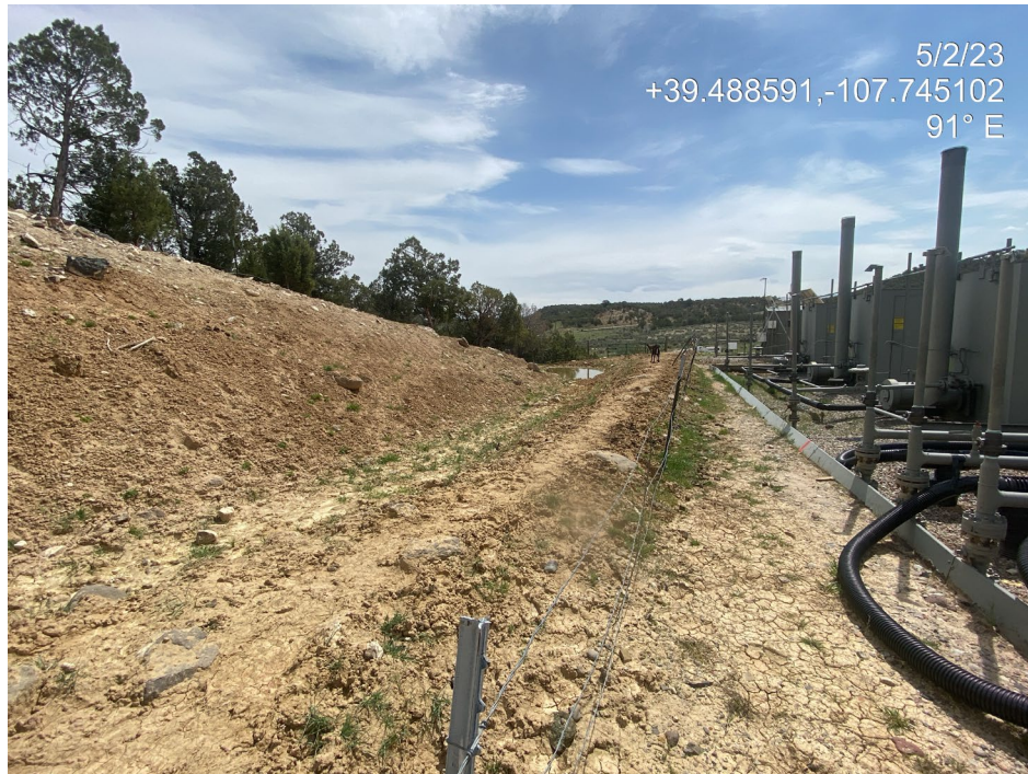
Photo 6. Photos show slopes to the northeast of the location lack stabilization.
