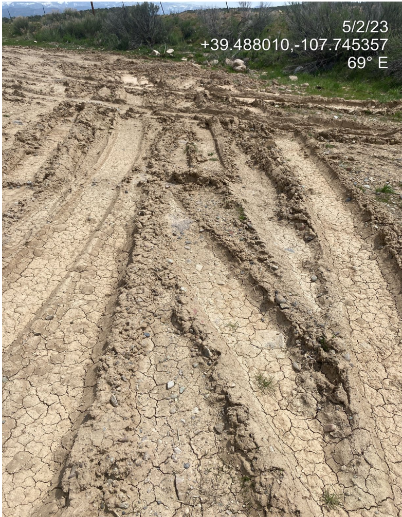
Photo 3. Photos show lack of stabilization of the pad surface to the south.
