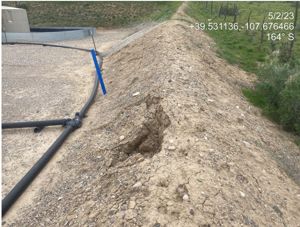
Photo 8. Photos show a berm to the west is unstabilized. Stormwater is traveling through the berm from the east (left) to the west (right).
