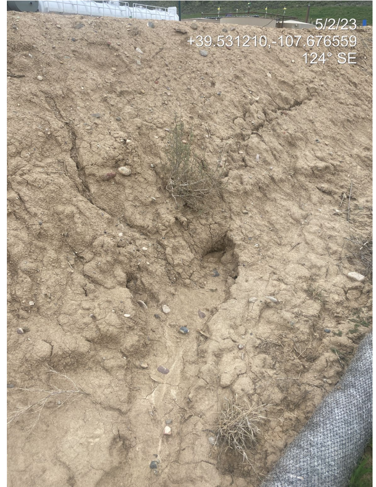
Photo 8. Photos show a berm to the west is unstabilized. Stormwater is traveling through the berm from the east (left) to the west (right).
