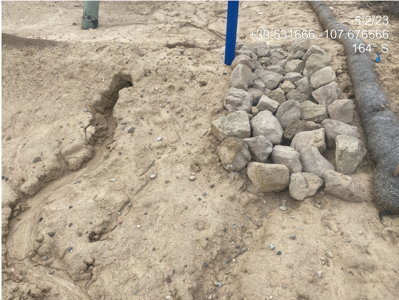
Photo 10. Photos taken to the northwest show stormwater is bypassing BMPs. Erosion degradation is evident.
