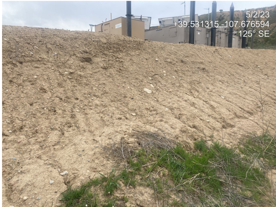
Photo 6. Photos show a berm to the west is unstabilized.
