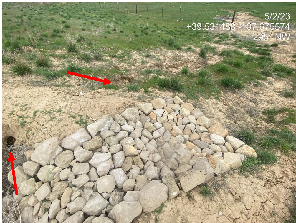
Photo 17. Photos show BMPs in the northern interim area of the location are not in proper functioning condition. Stormwater is bypassing the sediment trap outlet causing degradation.
