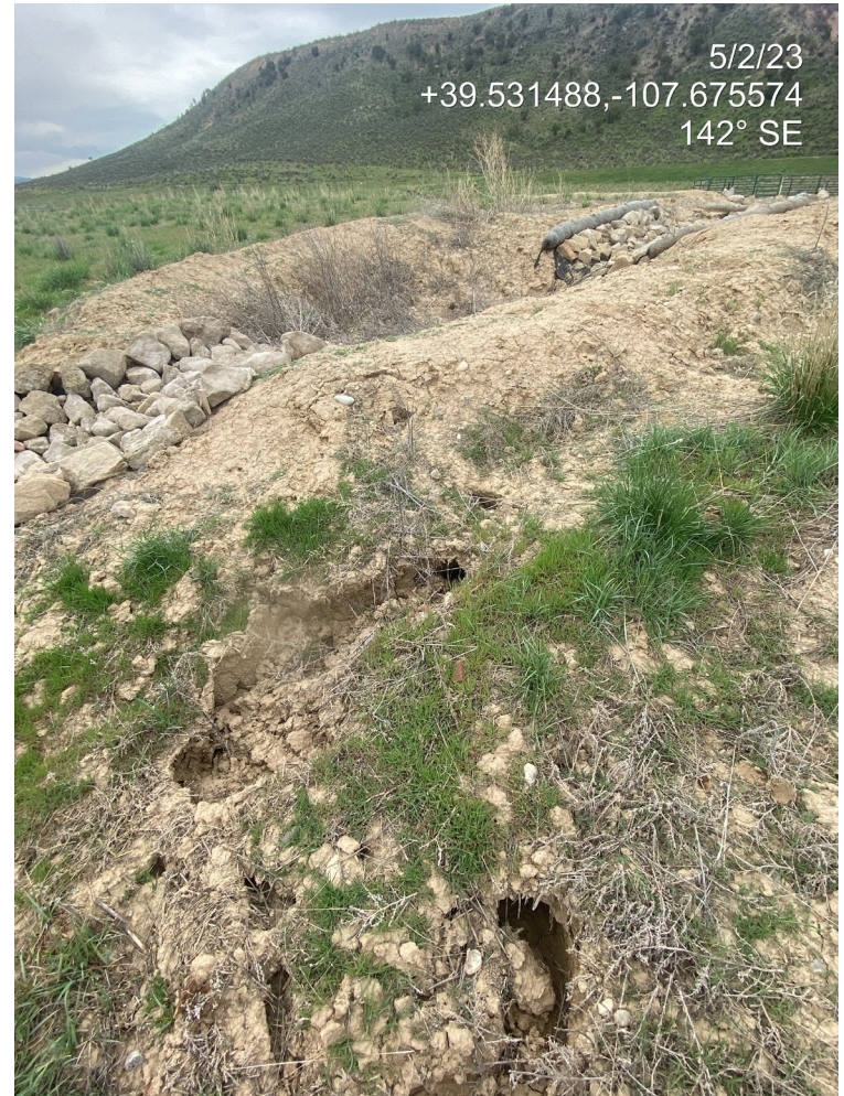
Photo 17. Photos show BMPs in the northern interim area of the location are not in proper functioning condition. Stormwater is bypassing the sediment trap outlet causing degradation.
