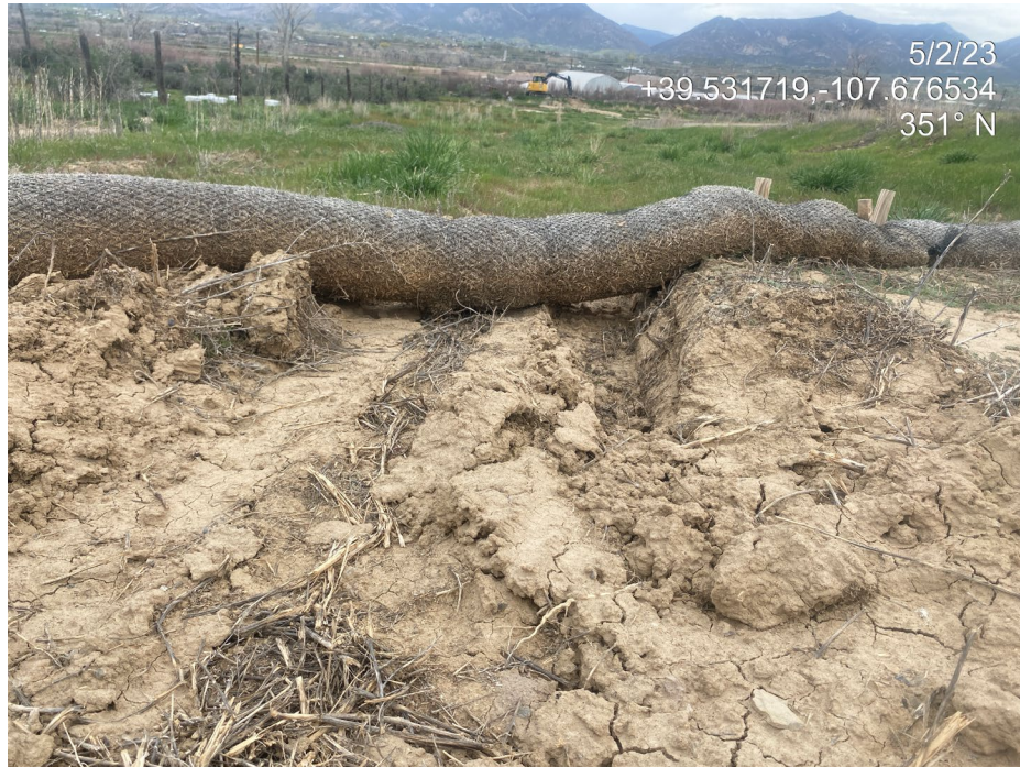
Photo 11. Photos taken to the northwest show BMPs not properly installed.
