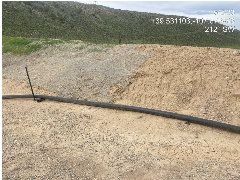
Photo 7. Photos show a berm to the west is unstabilized.
