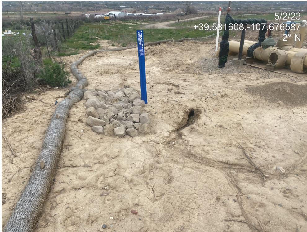
Photo 9. Photos taken to the northwest show stormwater is bypassing BMPs. Erosion degradation is evident.
