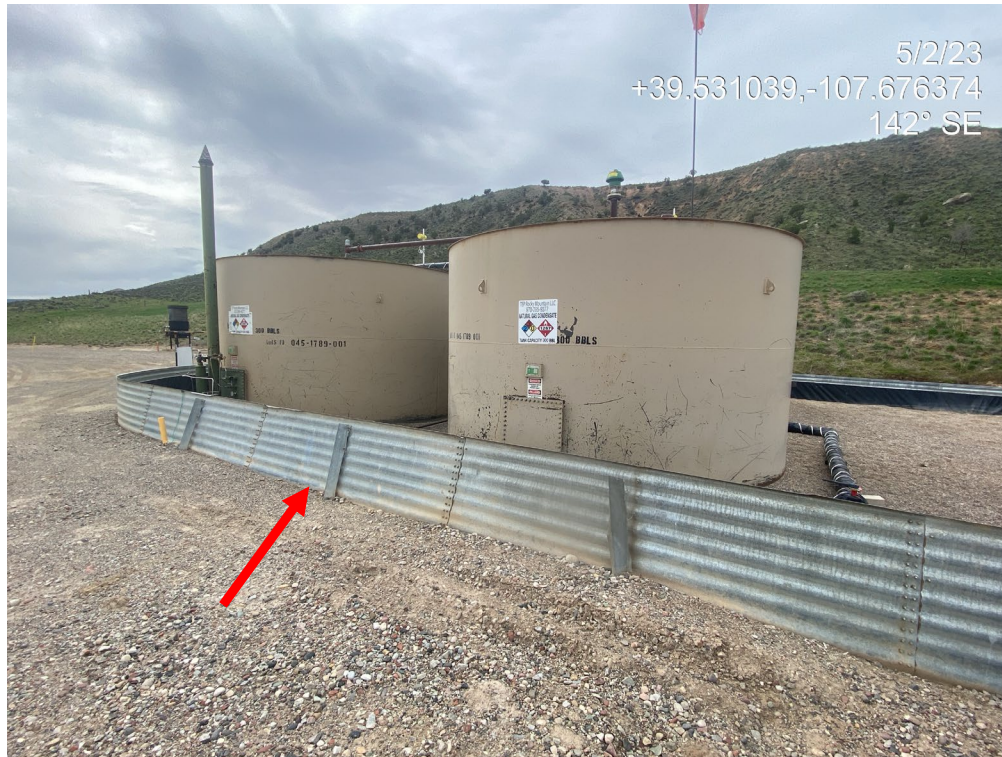
Photo 3. Photos show the tank secondary containment has been damaged (left) and an unmarked anchor (right).
