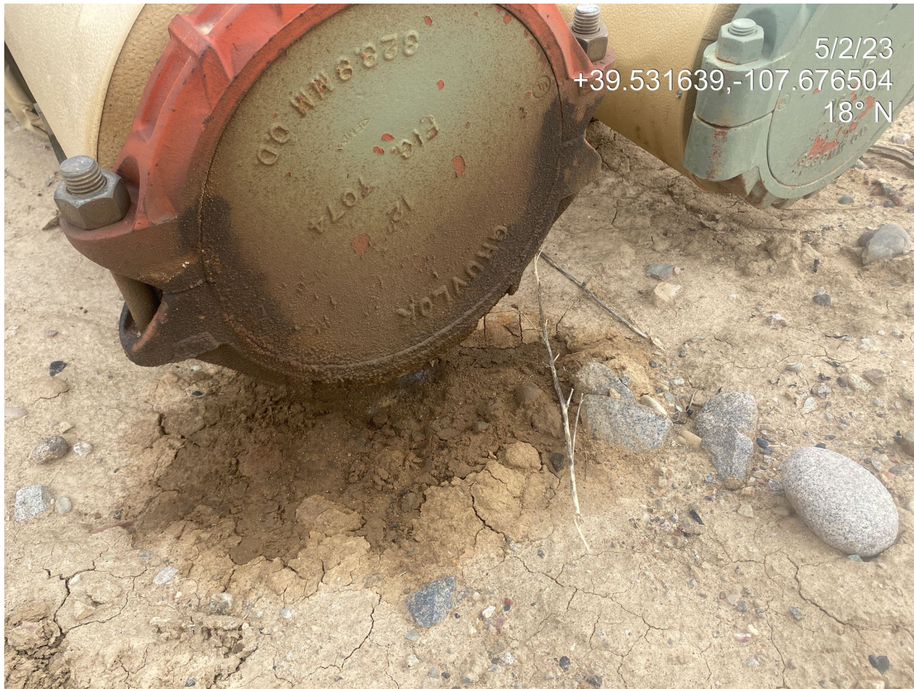
Photo 5. Photo shows staining at a pigging station to the northwest of the location.
