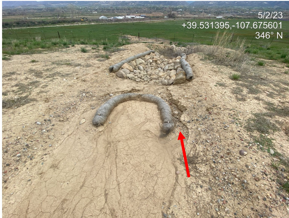
Photo 15. Photos show erosion degradation at stormwater BMPs in the northern interim area of the location.
