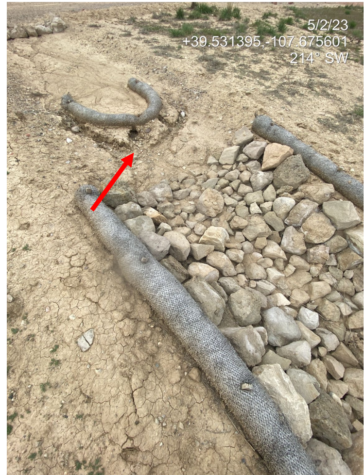
Photo 15. Photos show erosion degradation at stormwater BMPs in the northern interim area of the location.
