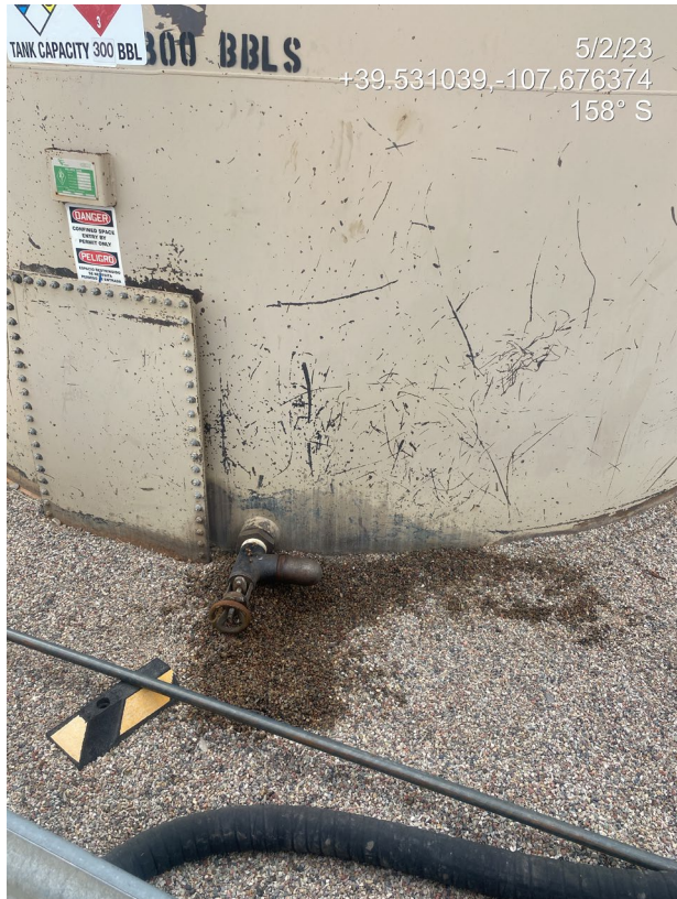
Photo 4. Photos show staining within the tank secondary containment.
