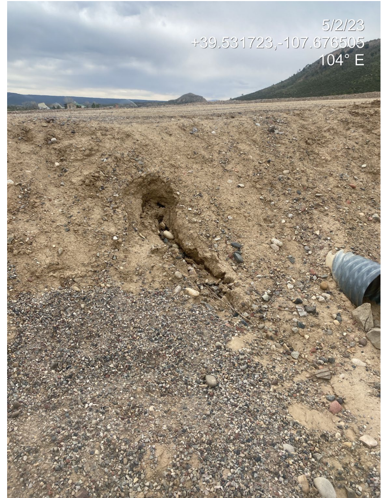
Photo 13. Photos taken to the northwest show where stormwater from the access road ditch is cutting through a berm (left) and exiting to the west (right).
