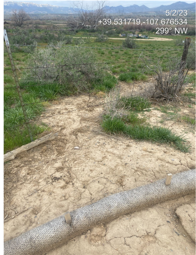
Photo 12. Photos taken to the northwest show erosion degradation migrating offsite downslope of BMPs and the unstabilized location.
