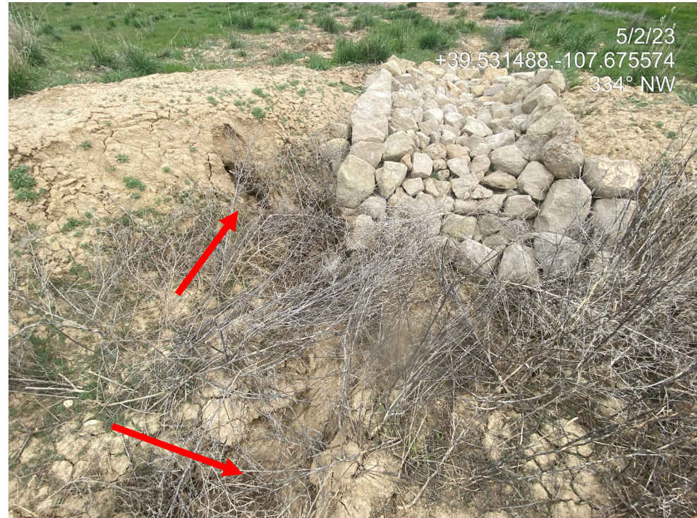
Photo 16. Photos show erosion degradation at stormwater BMPs in the northern interim area of the location. Stormwater is eroding the sediment trap at the inlet, (left) base and walls/outlet (right).
