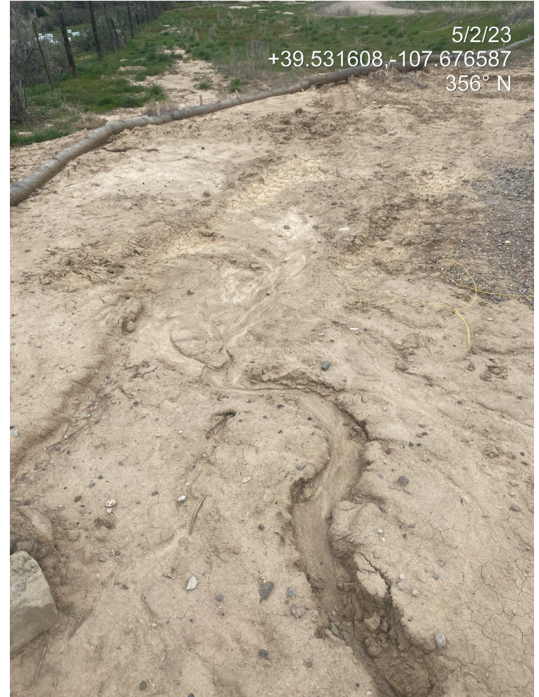
Photo 9. Photos taken to the northwest show stormwater is bypassing BMPs. Erosion degradation is evident.
