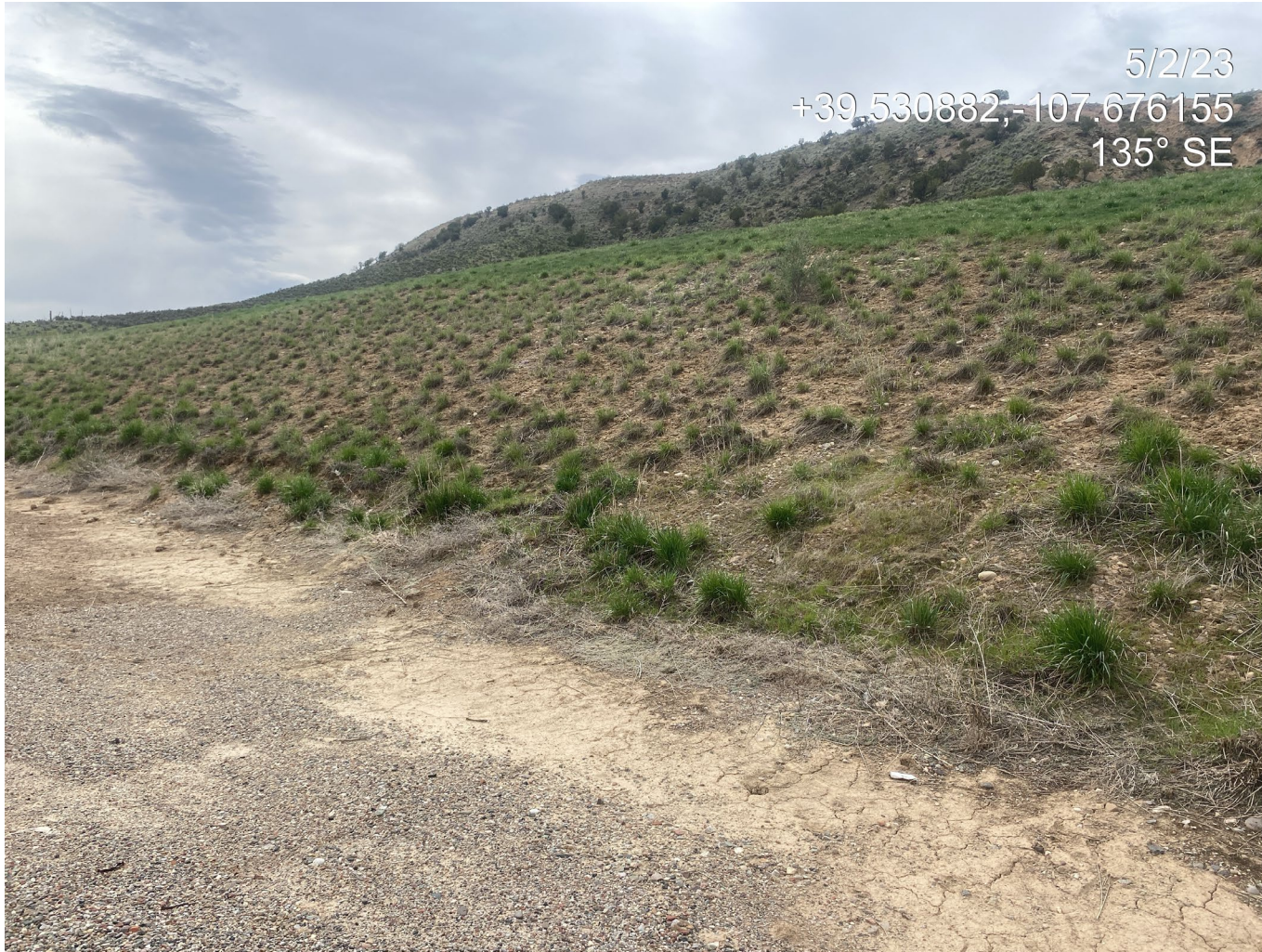
Photo 19. Photo shows a slope to the south stabilized by perennial grasses.
