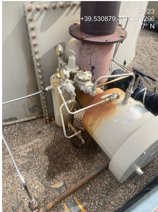
Photo 4. Photos show staining within the tank secondary containment.
