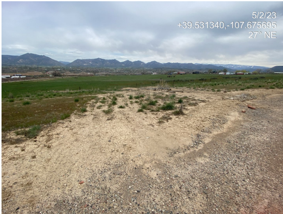
Photo 14. Photos show an overview of stormwater BMPs in the northern interim area of the location. Note lack of stabilizing perennial vegetation and sediment migration.
