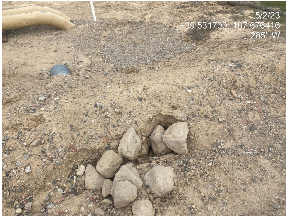
Photo 13. Photos taken to the northwest show where stormwater from the access road ditch is cutting through a berm (left) and exiting to the west (right).
