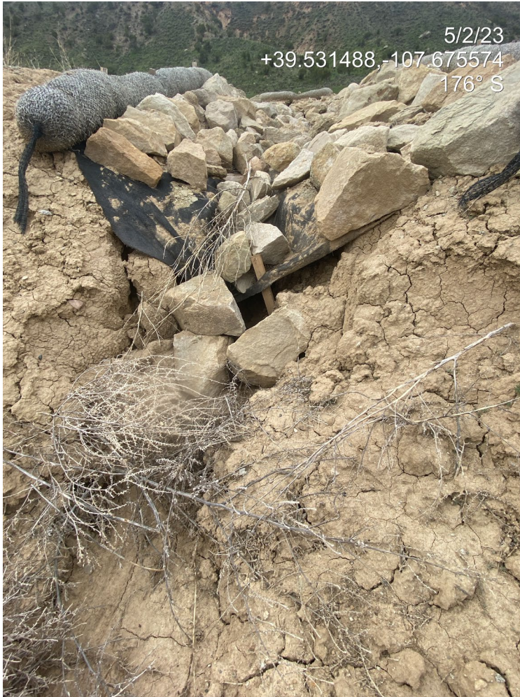
Photo 16. Photos show erosion degradation at stormwater BMPs in the northern interim area of the location. Stormwater is eroding the sediment trap at the inlet, (left) base and walls/outlet (right).
