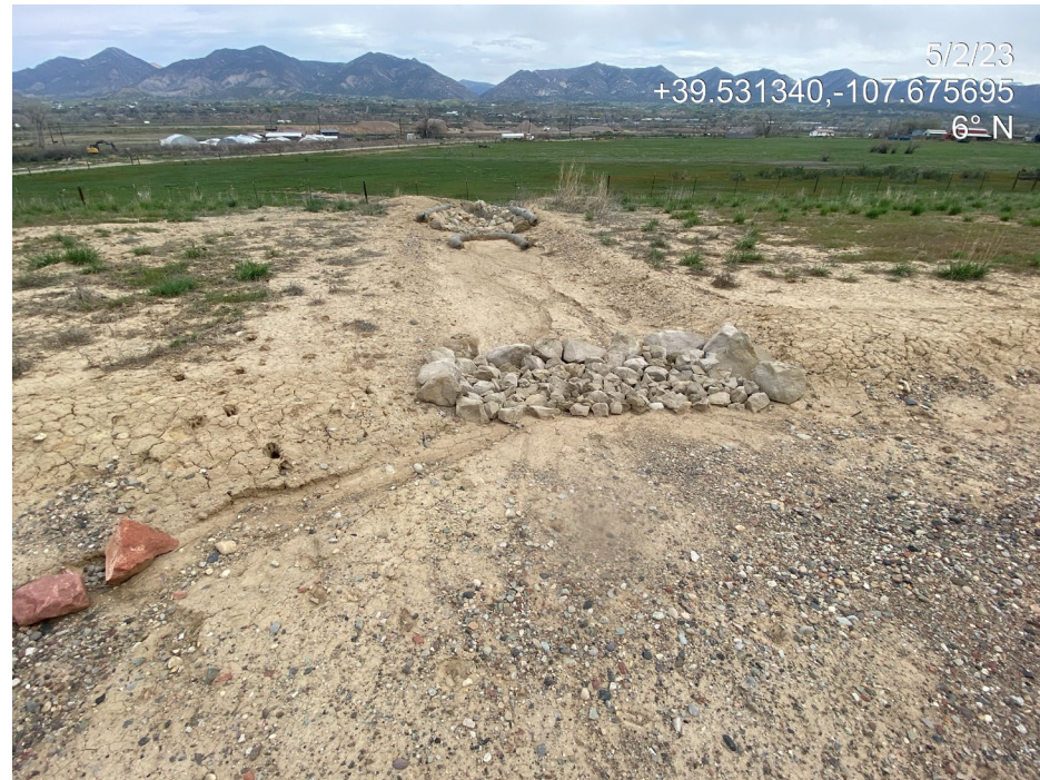
Photo 14. Photos show an overview of stormwater BMPs in the northern interim area of the location. Note lack of stabilizing perennial vegetation and sediment migration.
