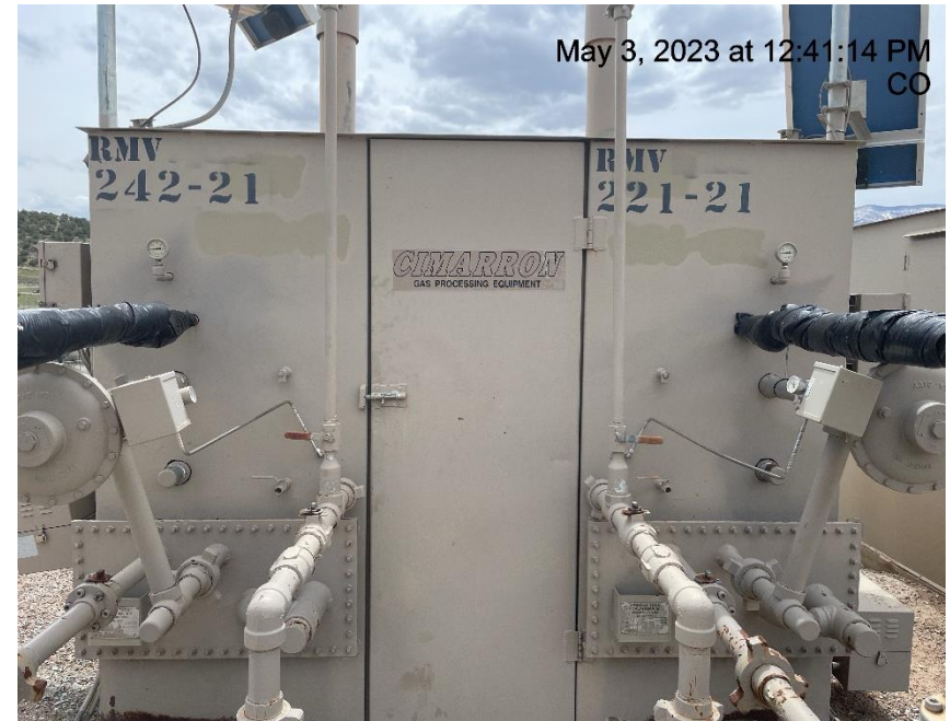
Photo # 6874 Meter calibration info not conspicuously posted
