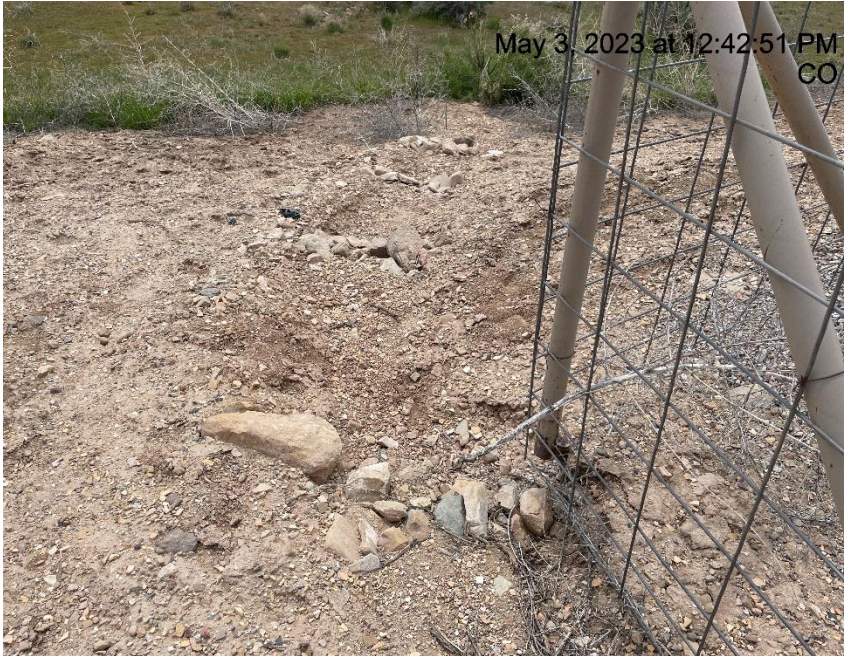
Photo # 6880 Check dams need maintenance
