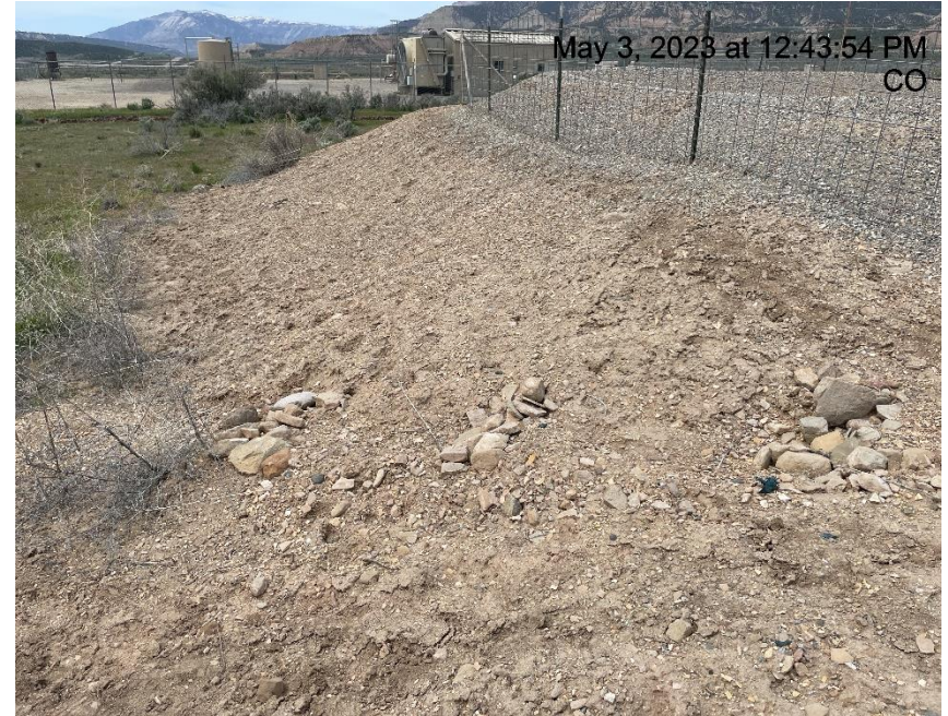
Photo # 6884 Check dams need maintenance
