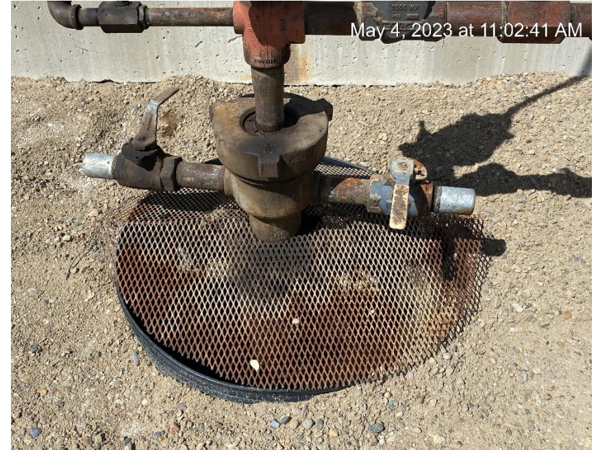
Bradenhead access below metal cover
