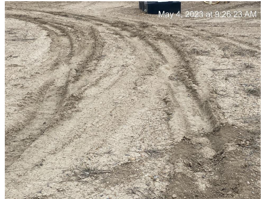
Lack of stabilization
