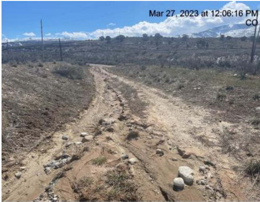
Photo # 3391 From Inspection 708900170 on 03/27/2023
