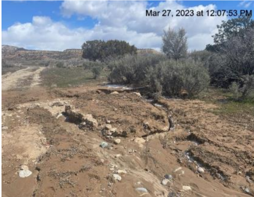
Photo # 3389 From Inspection 708900170 on 03/27/2023
