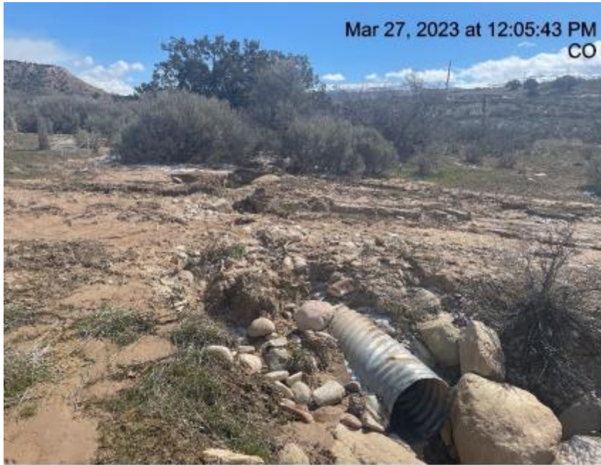
Photo # 3387 From Inspection 708900170 on 03/27/2023
