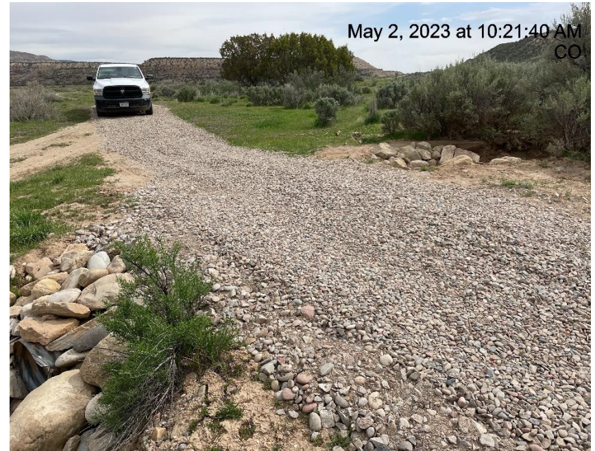
Photo # 6728 Repaired BMP's
