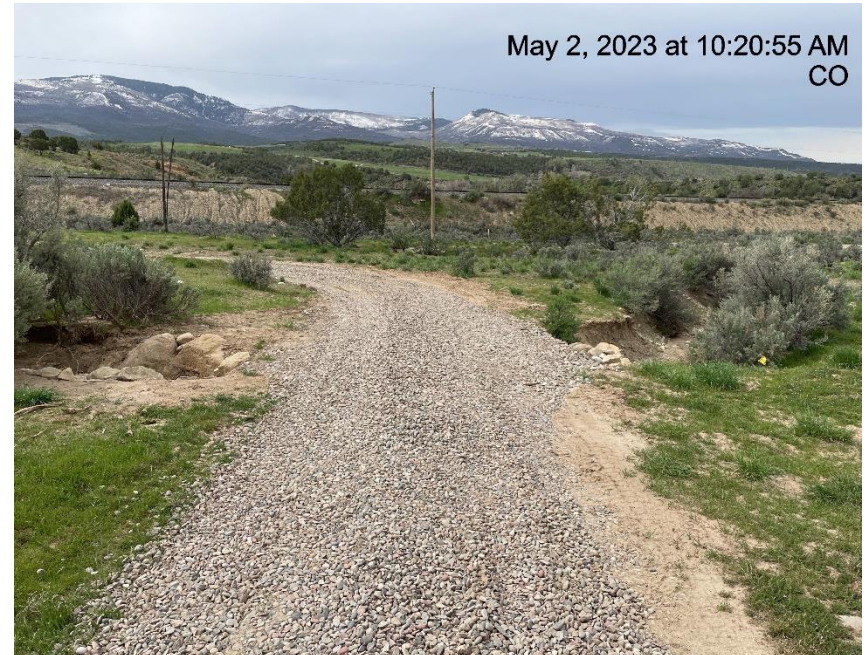
Photo # 6727 Repaired BMP's
