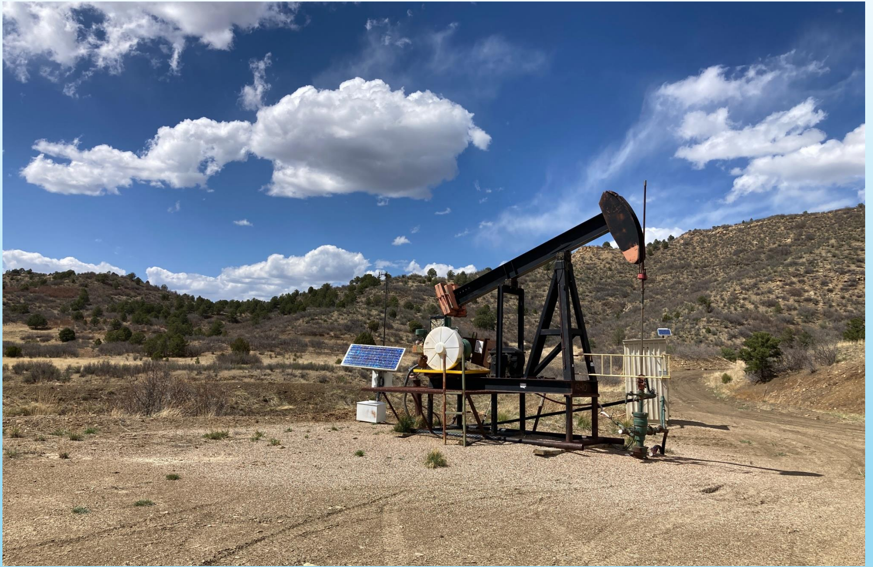
PHOTO 3: WELLHEAD AND EQUIPMENT
