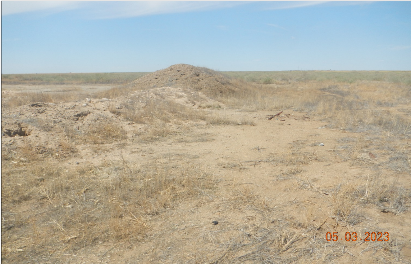
Photo 4. There are gravel and soil piles that remain at the north side of the location. The piles need to be removed. There are undesirable weeds on the piles.
