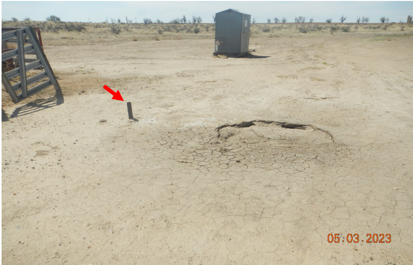
Photo 4. This is the area the broken tank was at. There is an uncapped pipe riser at the red arrow that likely fed into the tank which need to be removed.
