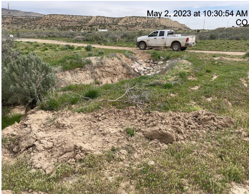
Photo # 6735 Stockpiled soils/insufficient BMP's, Soils/sediment choking off vegetation
