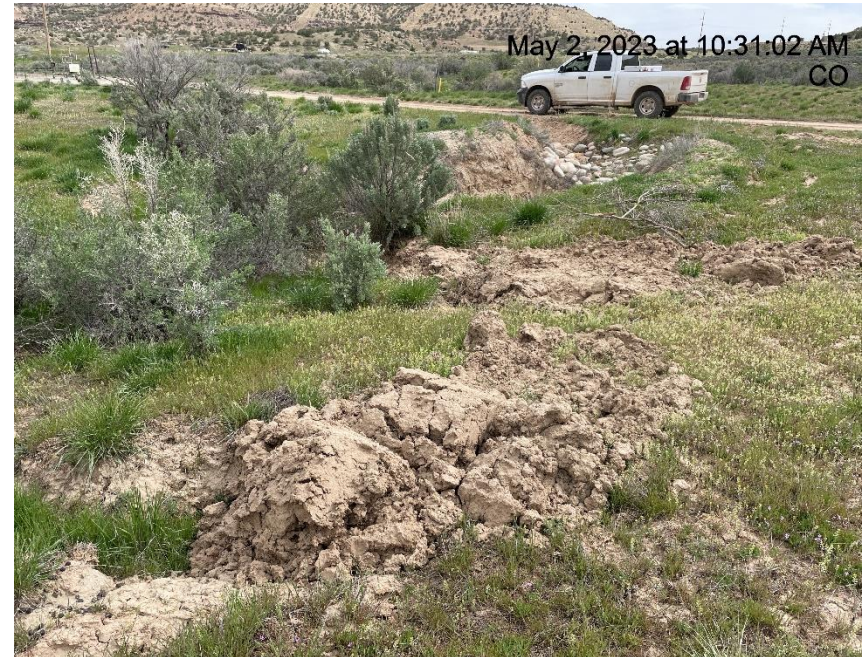
Photo # 6736 Stockpiled soils/insufficient BMP's, Soils/sediment choking off vegetation
