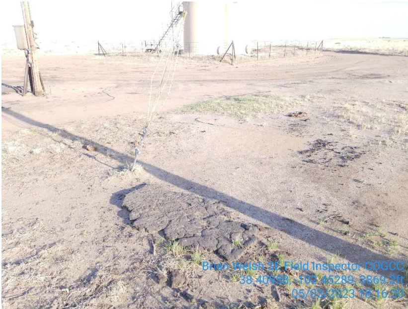
5. The west power pole has this stained soil on the east side of it
