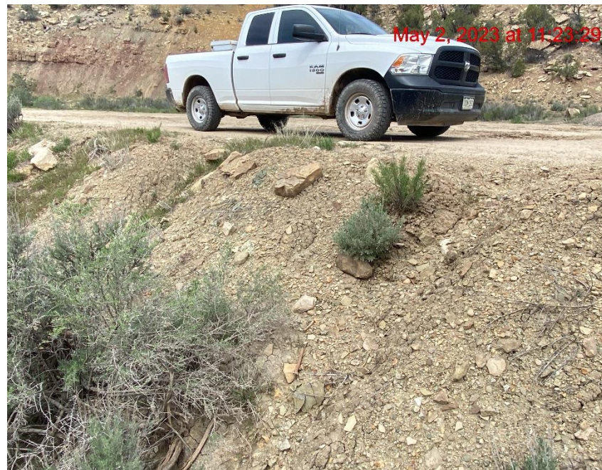
Sediment Transport from Access Road to Drainage Ditch – Photo #02759
