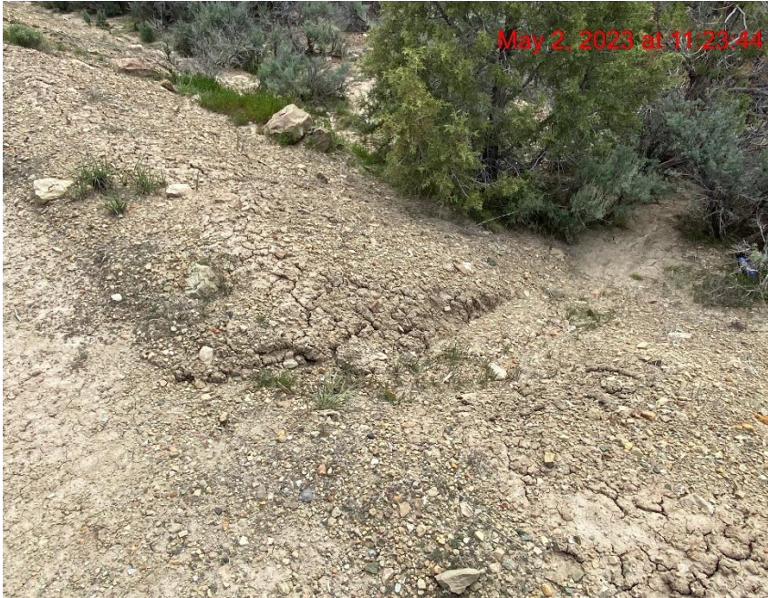
Sediment Transport from Access Road to Drainage Ditch – Photo #02760
