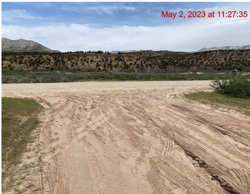
Insufficient Vehicle Tracking BMPs at Location Entrance/Exit – Photo #02766
