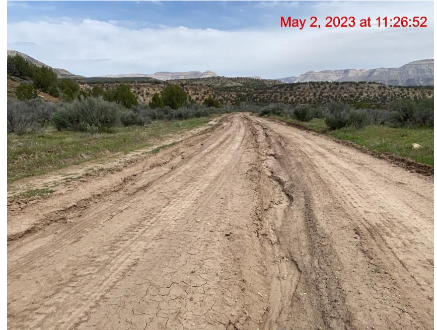
Rill Erosion on Access Road/Lack of Stabilization – Photo #02765
