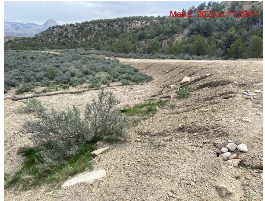
Rill Erosion Transporting Sediment from Location – Photo #02752
