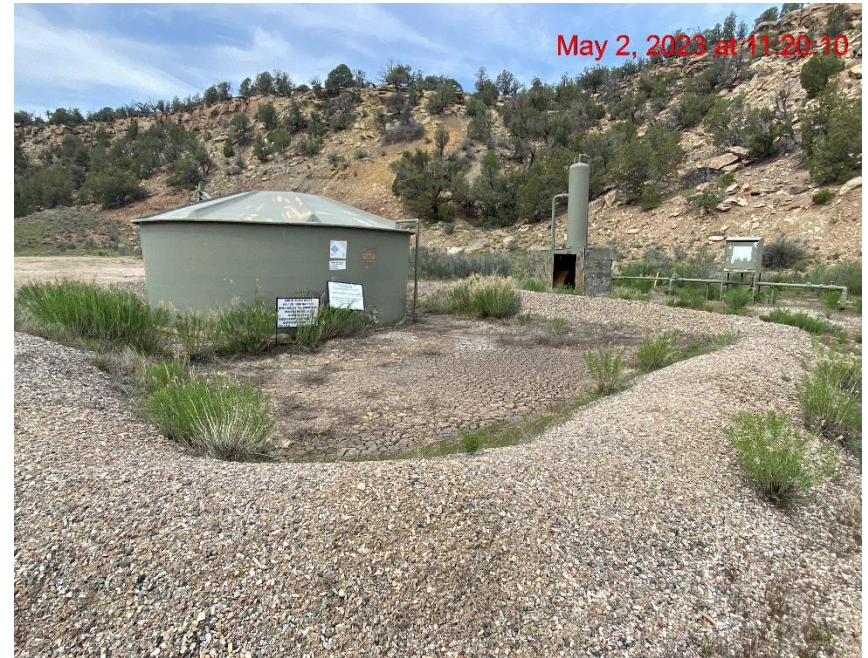
Tank Berm Permeability Insufficient due to Weed Growth – Photo #02750
