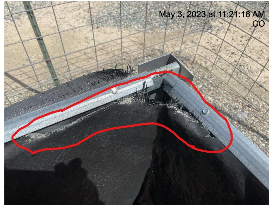
Photo # 6800 Containment needs maintenance
