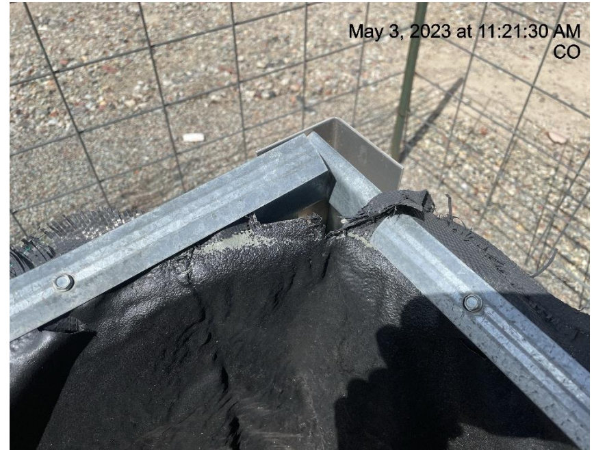
Photo # 6801 Containment needs maintenance
