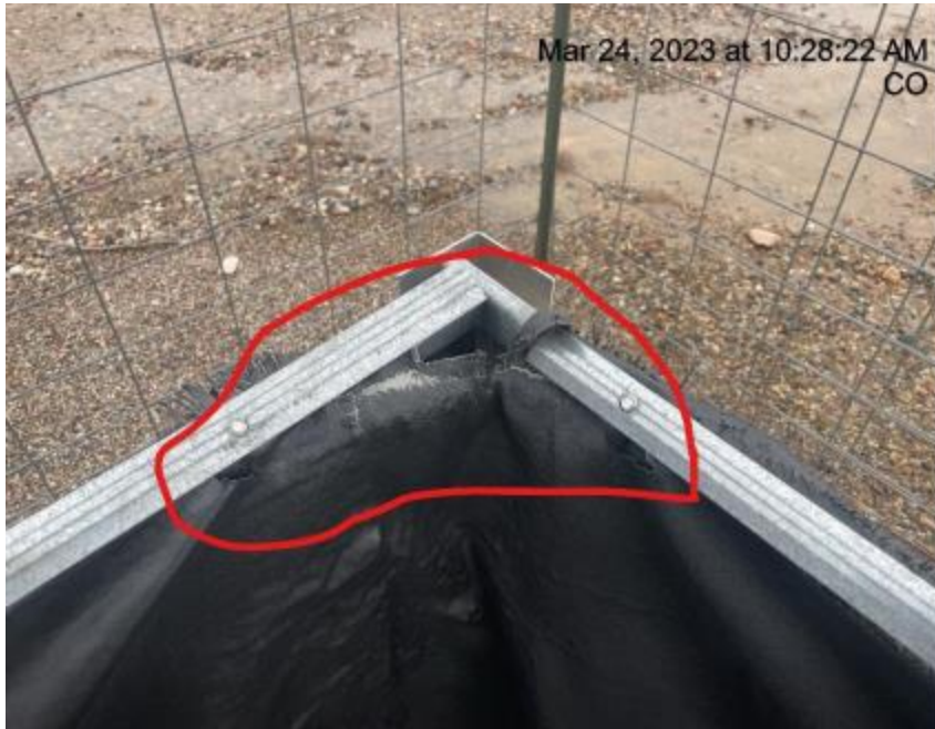
Photo # 3119 From Inspection 708900164 conducted on 03/24/2023 Containment needs maintenance
