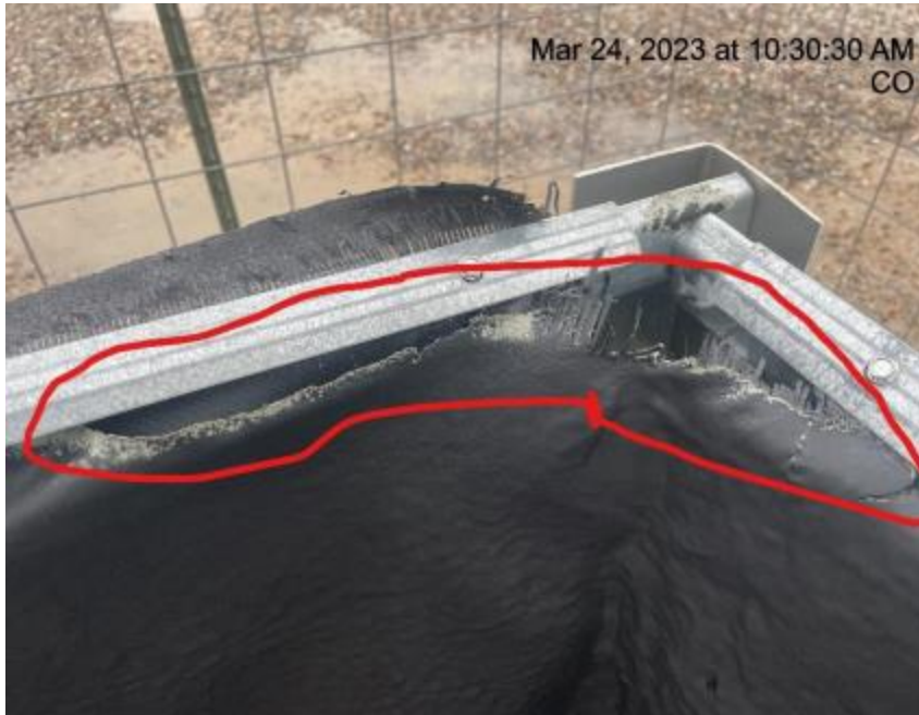
Photo # 3120 From Inspection 708900164 conducted on 03/24/2023 Containment needs maintenance
