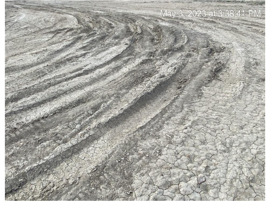
Lack of stabilization. No vehicle tracking pads
