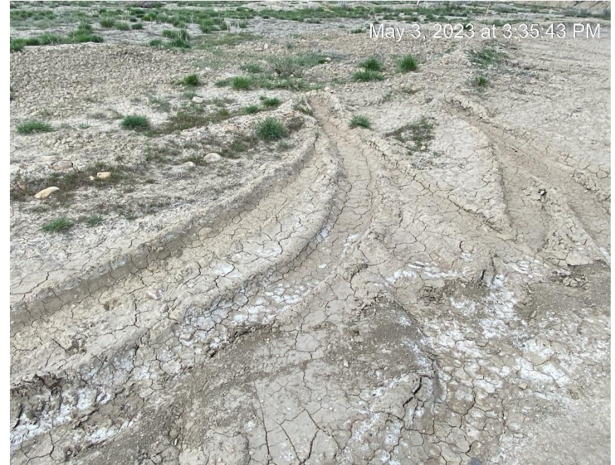
Lack of stabilization. Vehicle tracking
