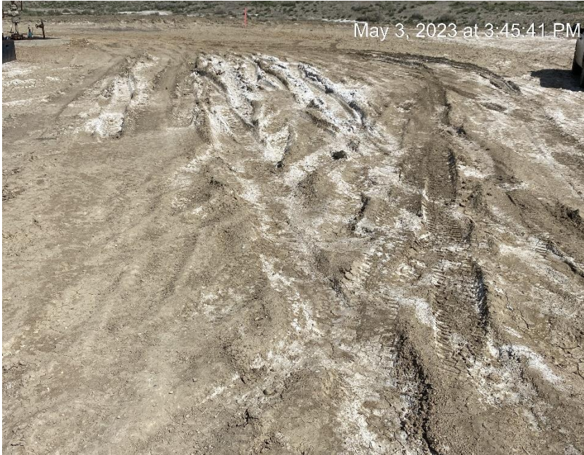
Lack of stabilization. No vehicle tracking pads
