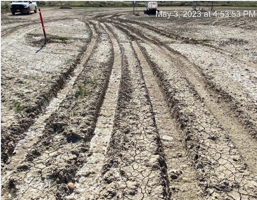
Lack of stabilization. No vehicle tracking pads
