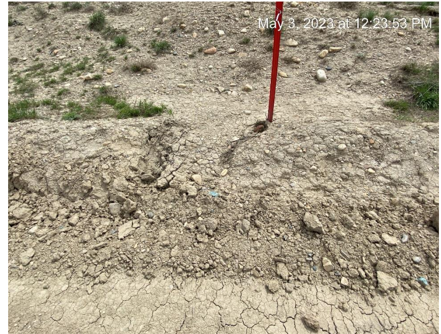
Slope erosion and sediment migration
