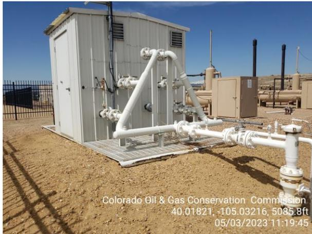
**Photo 15 Gas Meter Run, pig station.**
