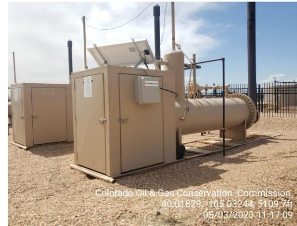
**Photo 14 Horizontal Heated separators.**
