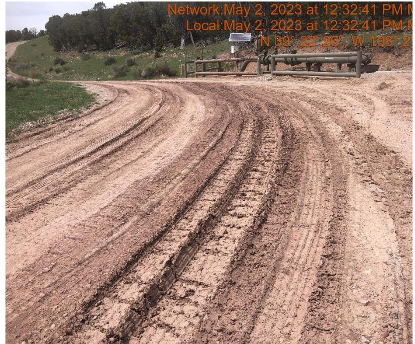
Photo #9811 Insufficient track BMP at entrance to location to minimize the transport of sediment.
