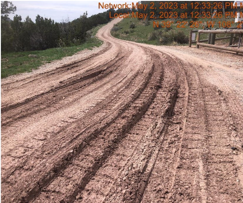
Photo #9814 Insufficient track BMP at entrance to location to minimize the transport of sediment.
