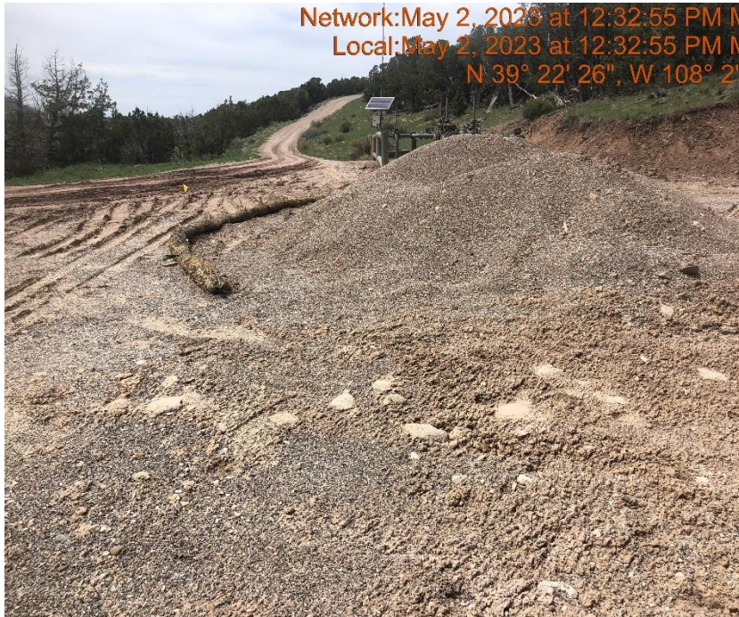
Photo #9812 Insufficient stockpiled soils BMP's.
