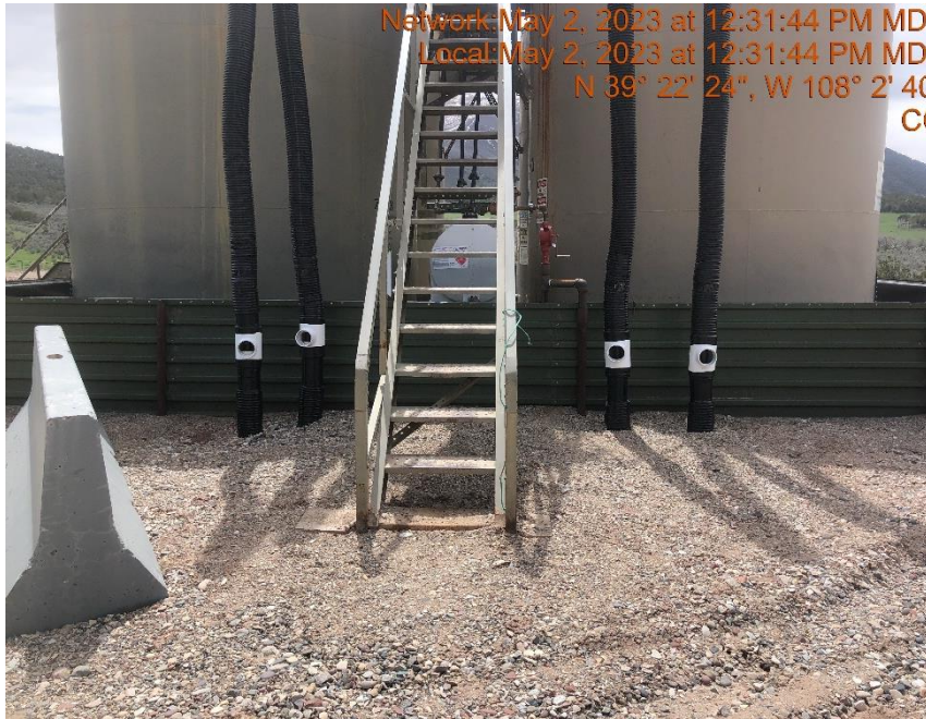
Photo #9809 Multiple flowline heating insulation open ended.
