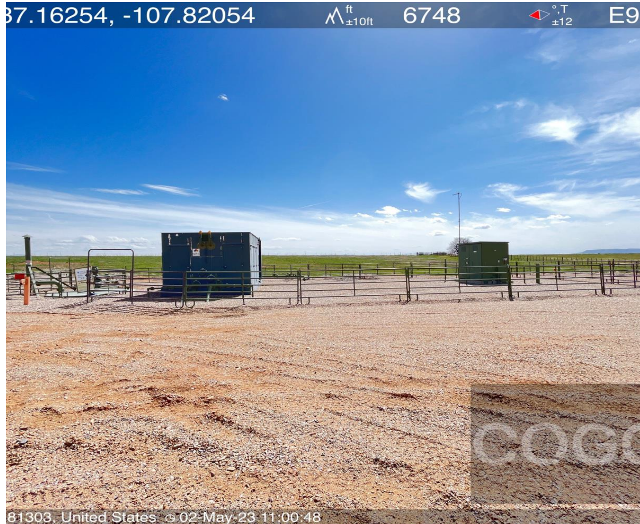
Photo #2. View of tank, separator, and meterhouse.
