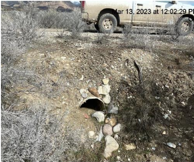
Photo # 2223 From Inspection 708900108 conducted on 03/13/2023 Culvert needs maintenance
