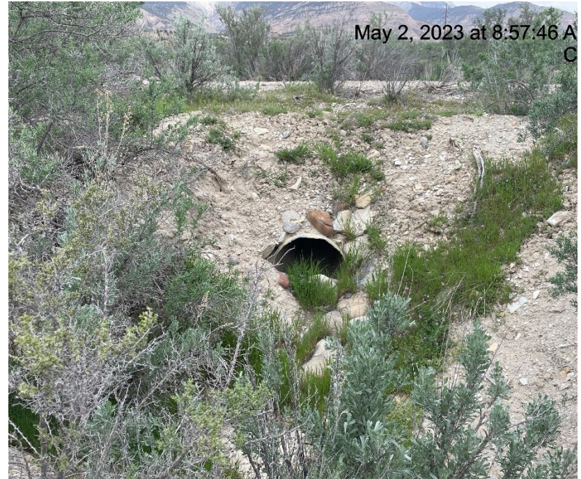
Photo # 6669 Culvert needs maintenance
