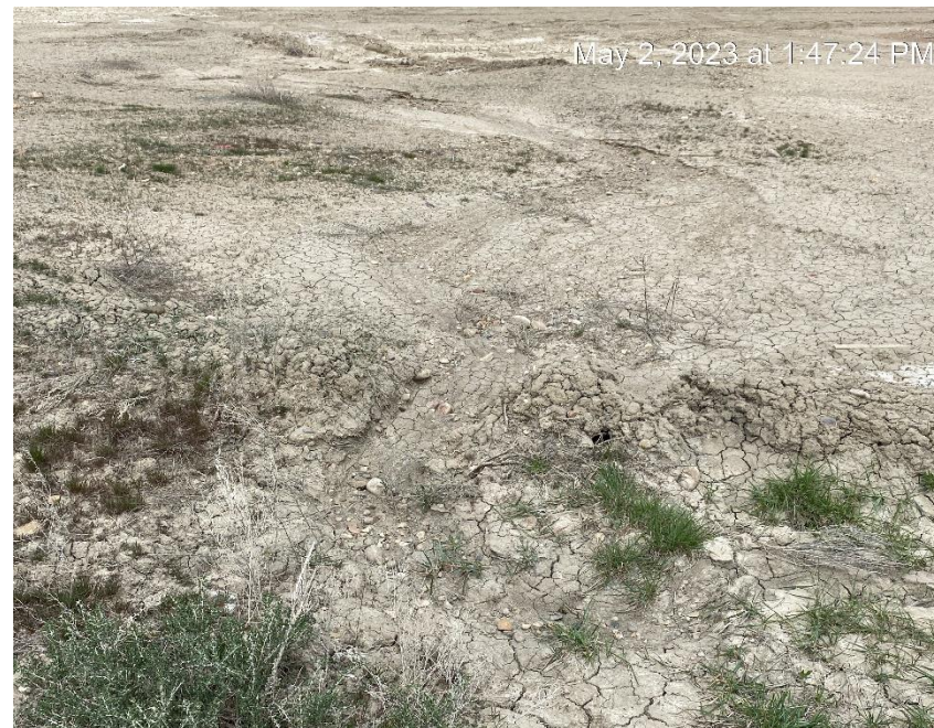
Sediment migration from diversion ditch
