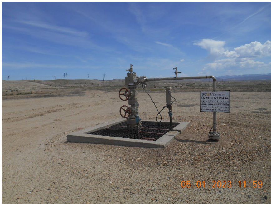
Injection wellhead
