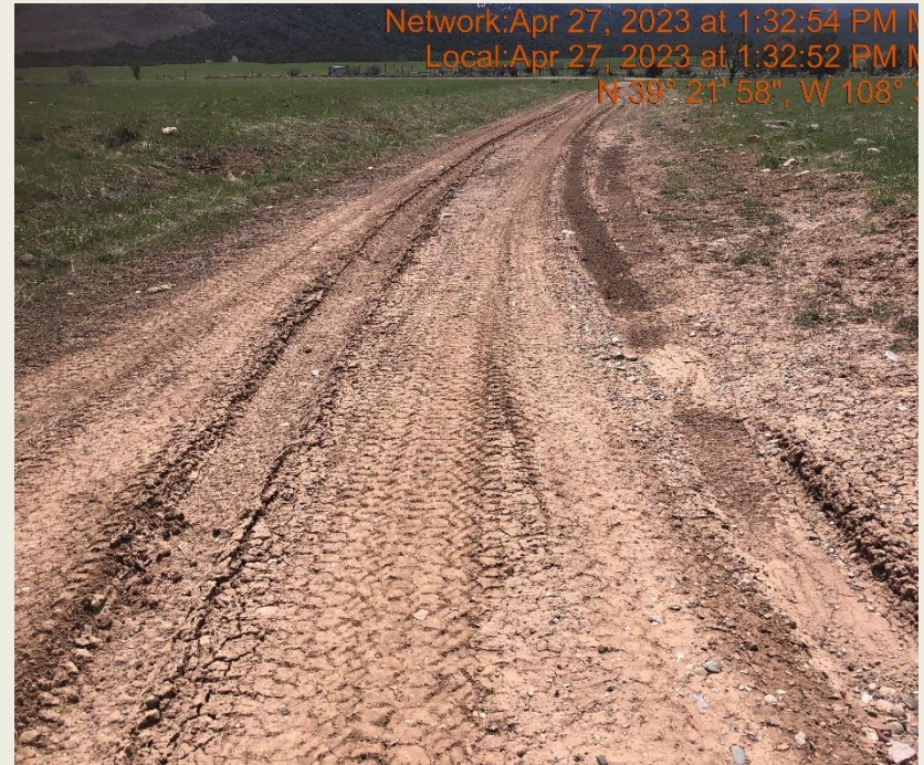
Photo #9786 Access road lacks stabilization.
