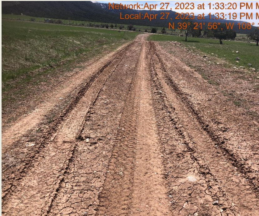
Photo #9788 Access road lacks stabilization.
