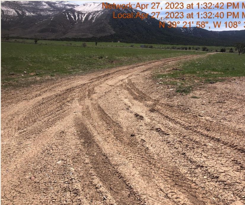
Photo #9785 Access road lacks stabilization.
