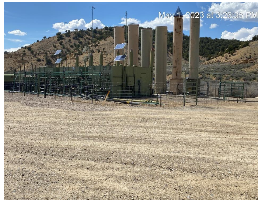
Separators and tank battery ECDs
