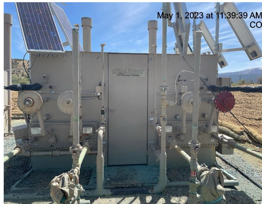
Photo # 6632 Meter calibration info not conspicuously posted
