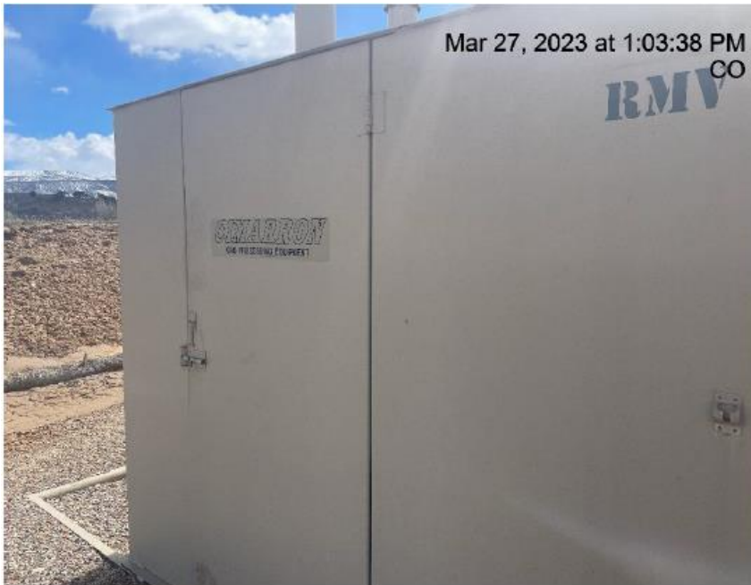
Photo # 3429 From Inspection 708900178 conducted on 03/27/2023 Meter calibration info not conspicuously posted
