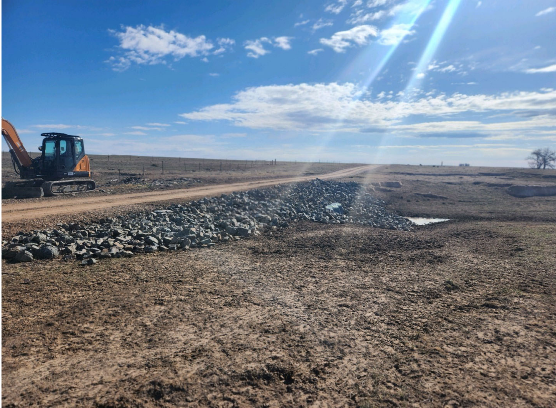
Rock checks were added alongside the lease road on the Southwest side and one location on the Northwest side to mitigate erosion issues
