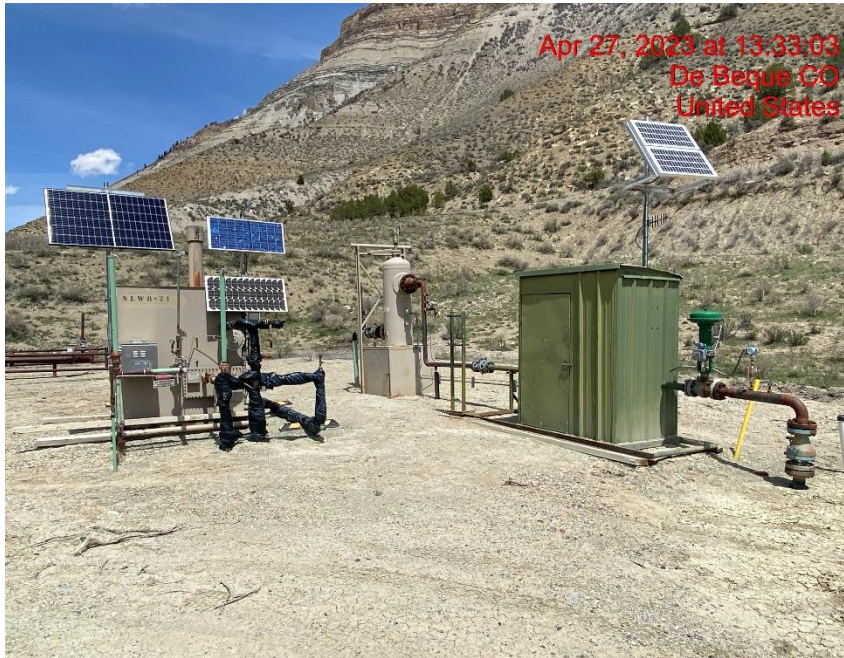
Separator/Gas Meter – Photo #02683
