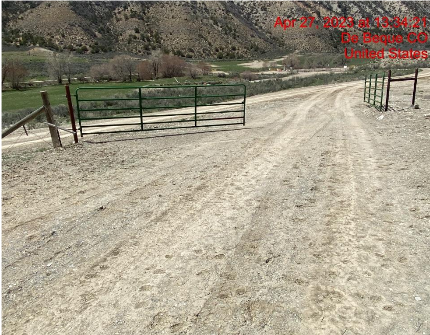
Insufficient Vehicle Tracking BMPs at Location Entrance/Exit – Photo #02686
