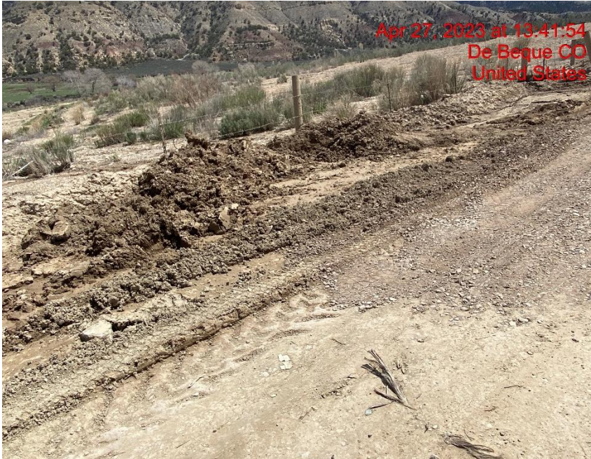
Lease Road Degradation/Transport of Sediment – Photo #02690
