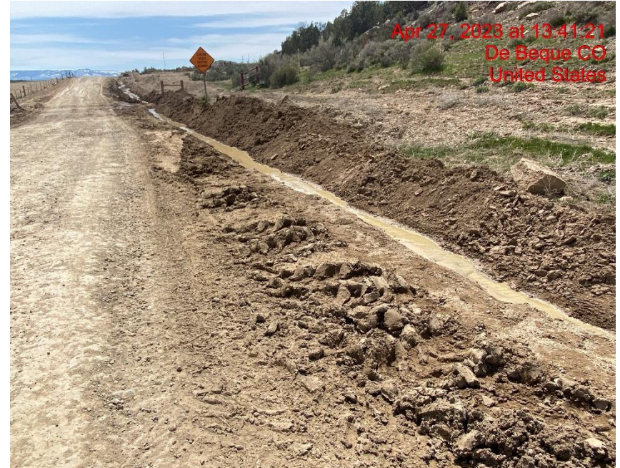
Lease Road Degradation/Transport of Sediment – Photo #02688
