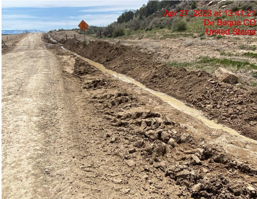
Lease Road Degradation/Transportation of Sediment – Photo #02688
