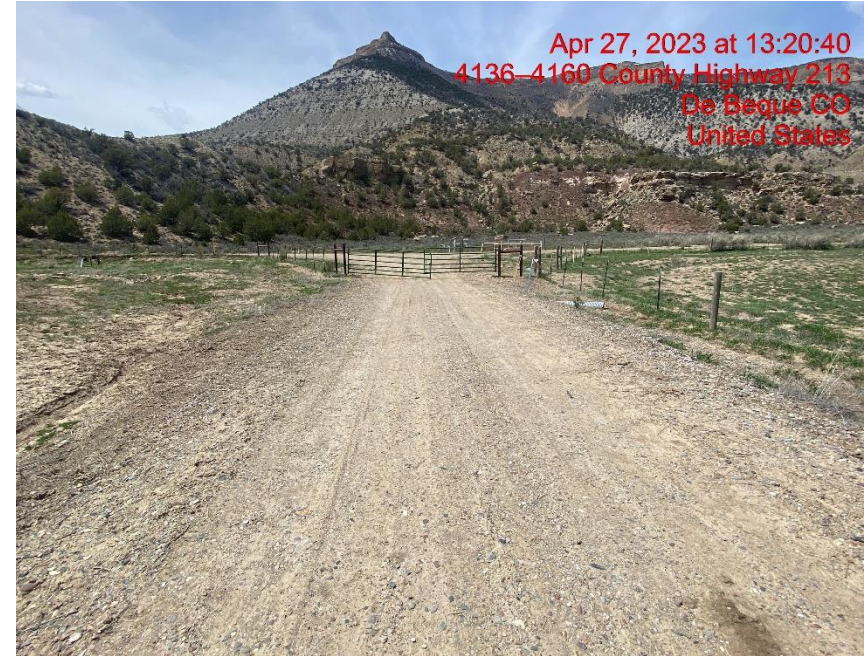
Insufficient Vehicle Tracking BMPs – Photo #02672
