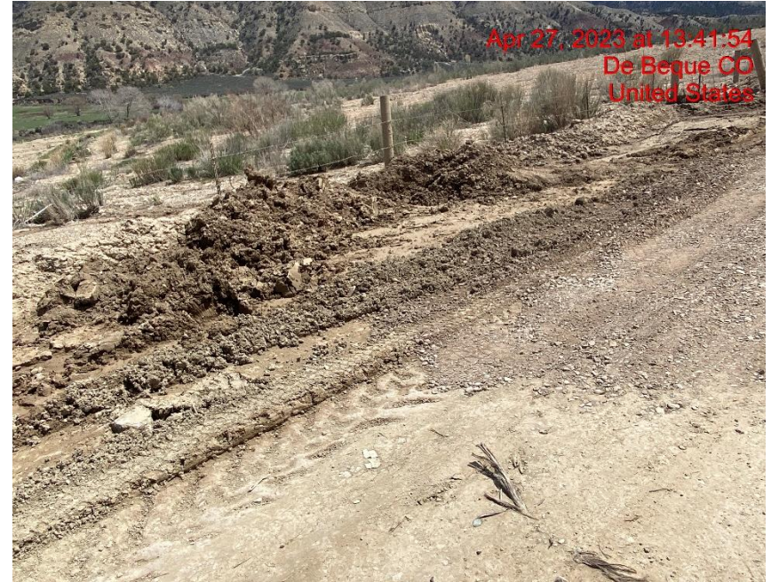
Lease Road Degradation/Transportation of Sediment– Photo #02690
