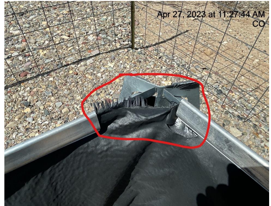
Photo # 6556 Containment liner needs maintenance
