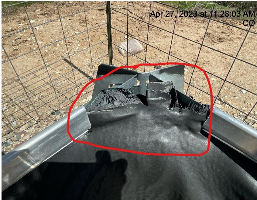
Photo # 6559 Containment liner needs maintenance
