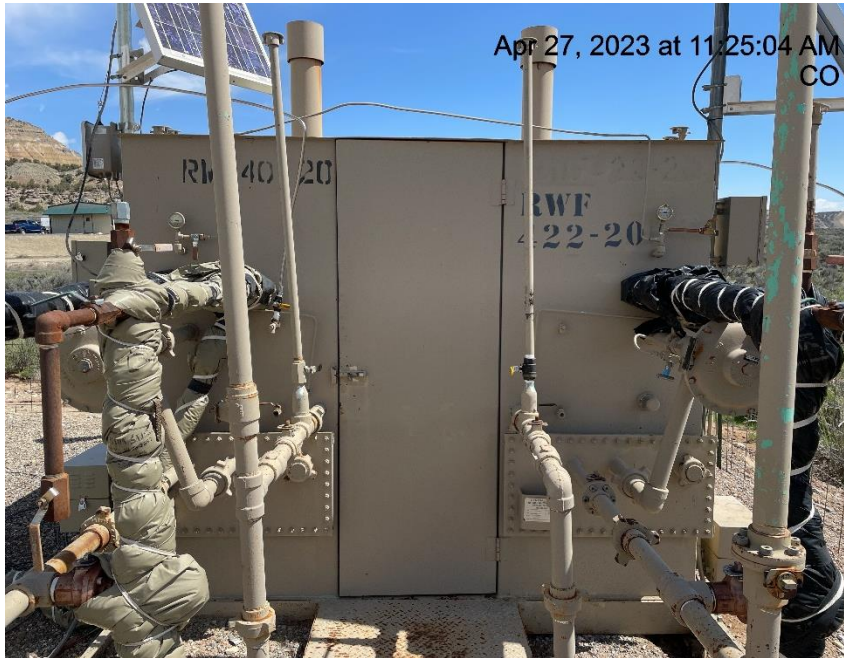
Photo # 6548 Meter calibration info not conspicuously posted
