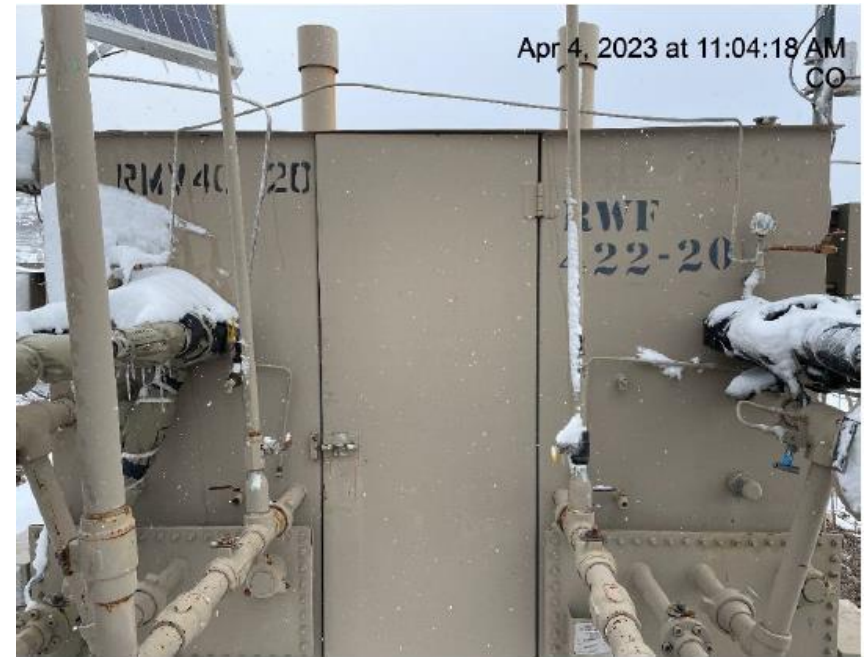
Photo # 4257 From inspection 708900217 conducted on 04/04/2023 Meter calibration info not conspicuously posted
