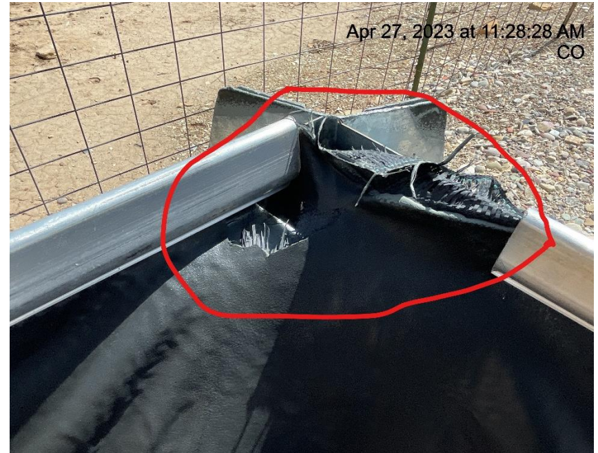
Photo # 6561 Containment liner needs maintenance
