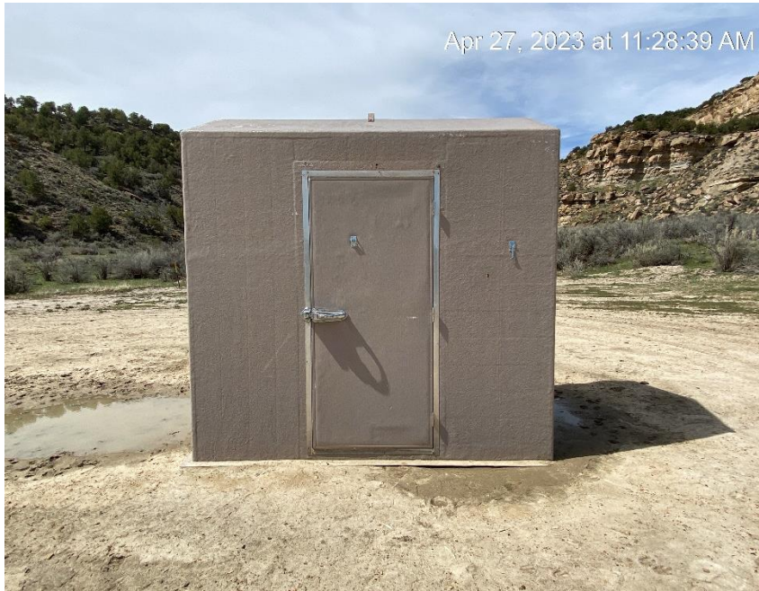
Fiberglass cover over wellhead
