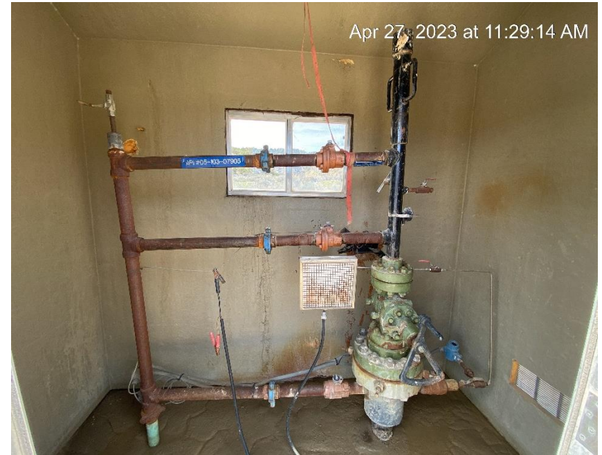
Wellhead inside wellhead cover
