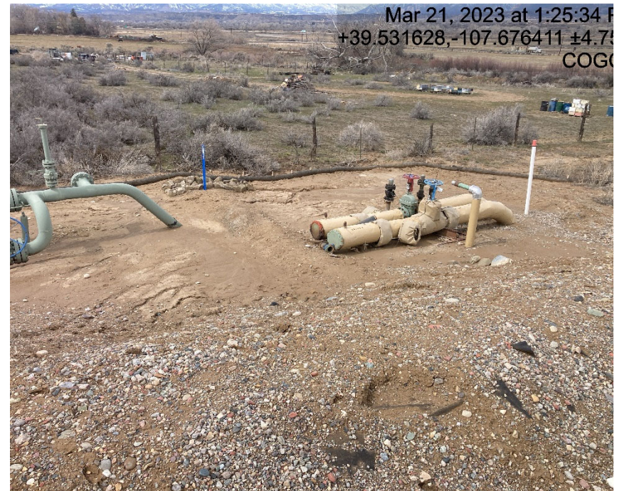
Photo from previous inspection of erosion and failing BMP's
