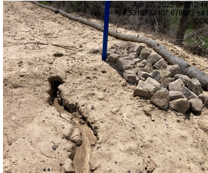
Erosion and tunneling next to rip rap
