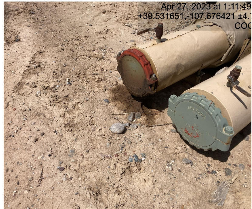
Staining next to all erosion and sediment migration
