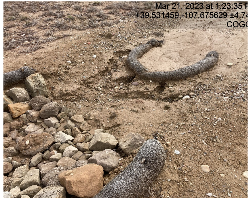
Erosion under waddles. Photo from previous inspection
