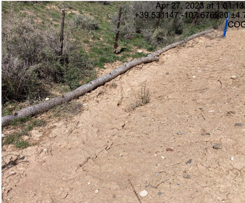
Fill slope shows lack of stabilization, Photo from Follow up inspection
