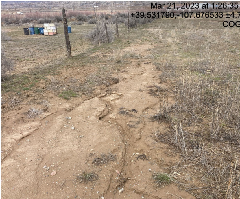
BMP's Failing and erosion channels with sediment migration. Photo from previous inspection
