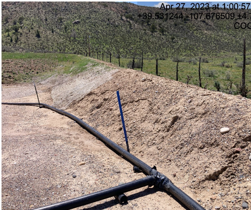
Berm shows signs of erosion. Photo from follow up inspection
