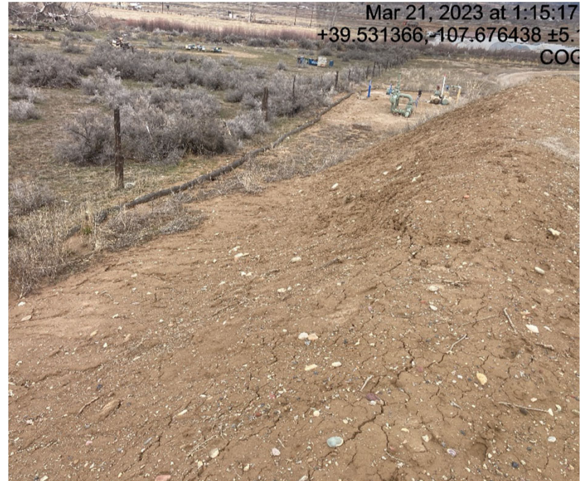
Fill slope shows lack of stabilization, Photo from previous inspection
