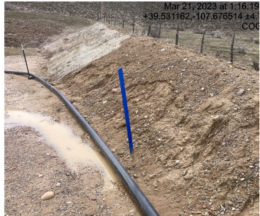
Berm shows signs of erosion. Photo from Previous inspection. Blankets have been installed in areas.
