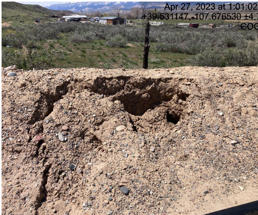
Erosion is undermining location berm coming out of fill slope. Photo from follow up inspection
