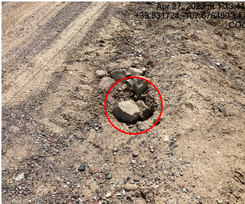
Tunneling through ditch at check dam out the side of the fill slope next to culvert
