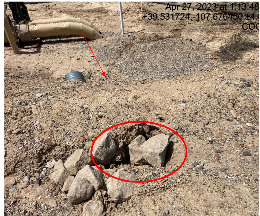
Tunneling through ditch at check dam out the side of the fill slope next to culvert. Circle is inlet and arrow is pointing to outlet.
