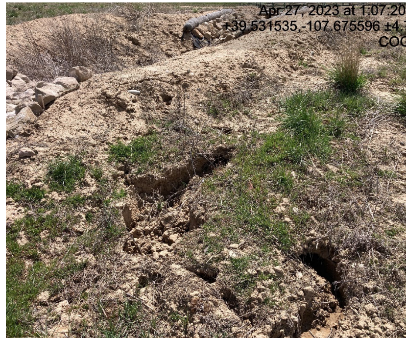
Outlet side of sediment trap tunneling and erosion channels with sediment migration
