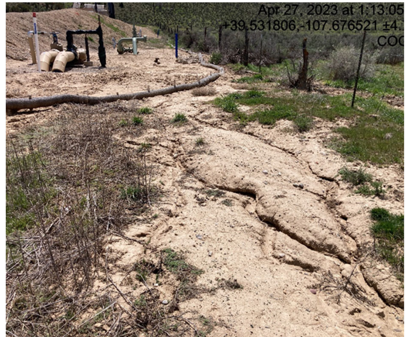
BMP's Failing and erosion channels with sediment migration. Photo from follow up inspection
