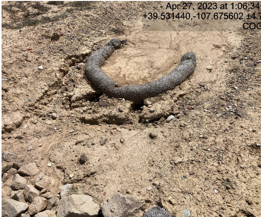
Erosion under waddles. Photo from follow up inspection
