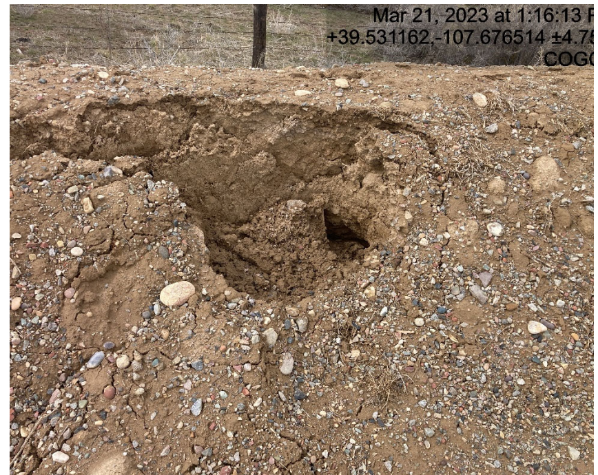
Erosion is undermining location berm coming out of fill slope. Photo from previous inspection
