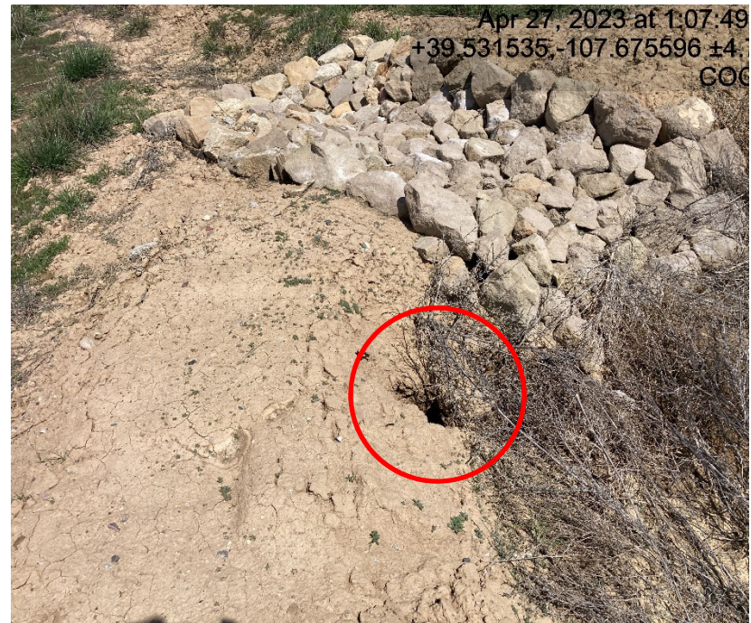
Circle indicates inlet of tunneling through sediment trap
