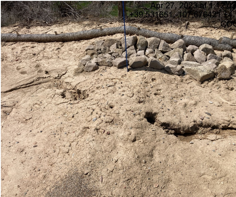
Erosion and tunneling next to rip rap
