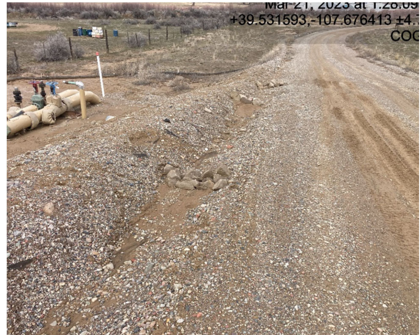
Access road BMP's Failing Photo from previous inspection
