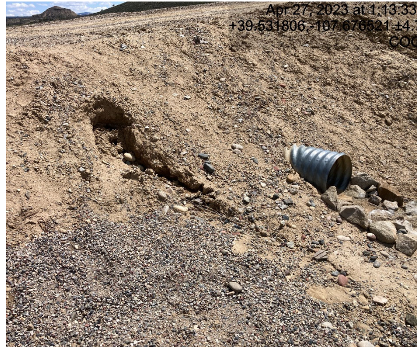
Outlet from tunneling occurring in access road ditch and erosion.
