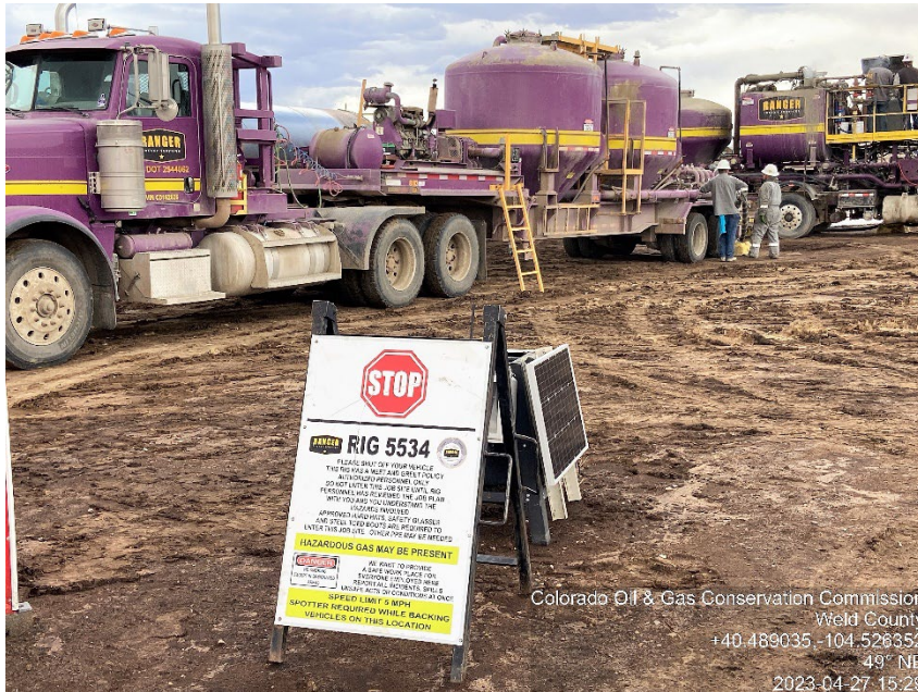
Photo #3 Rayglo A14-68-1HN Wellsite Plugged & Abandoned | PA Plugging Ops: Cementing: Final plugs / cement to surface Cementing Units
