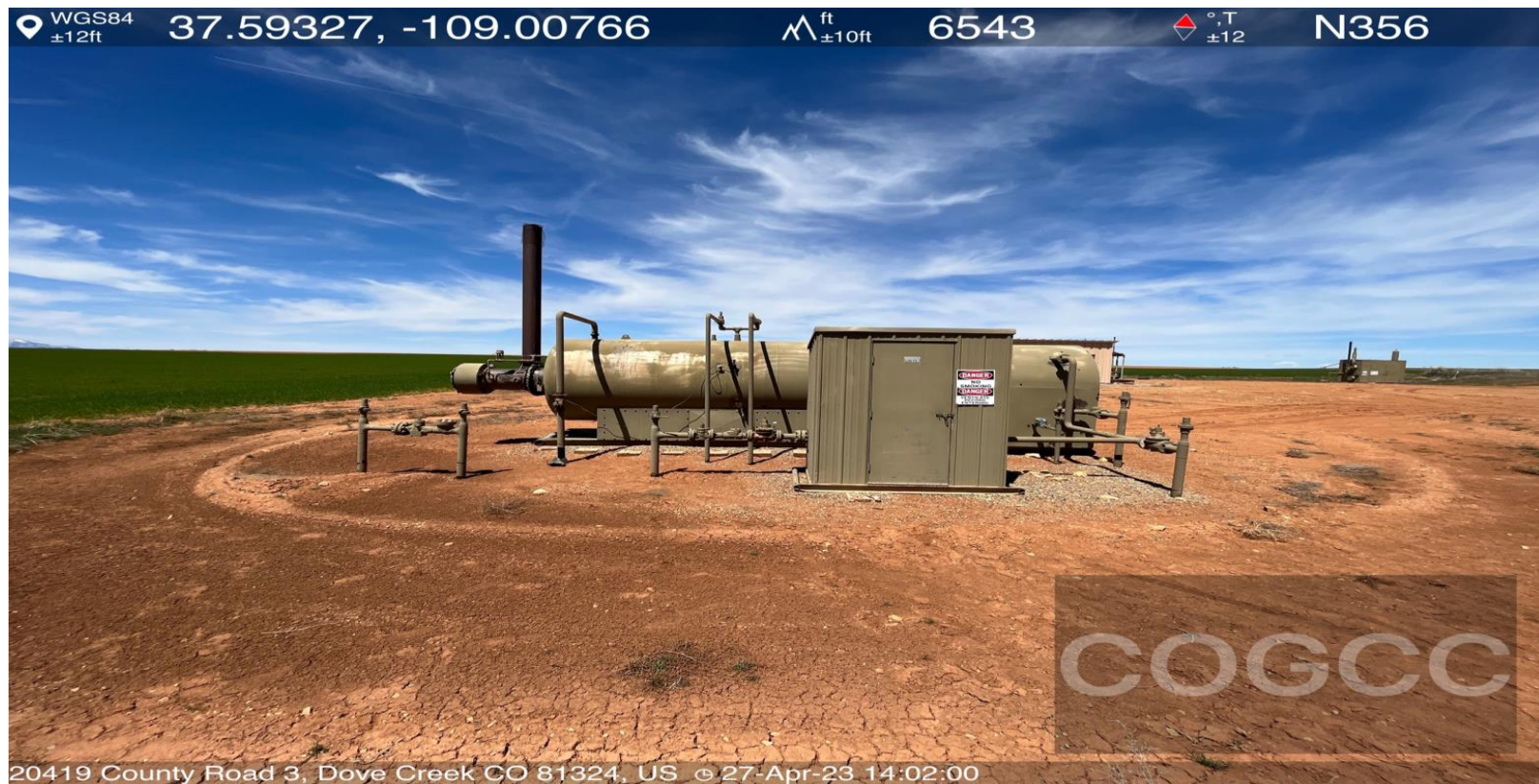
Photo #3. Horizontal separator (westside #1) eroded containment berm.
