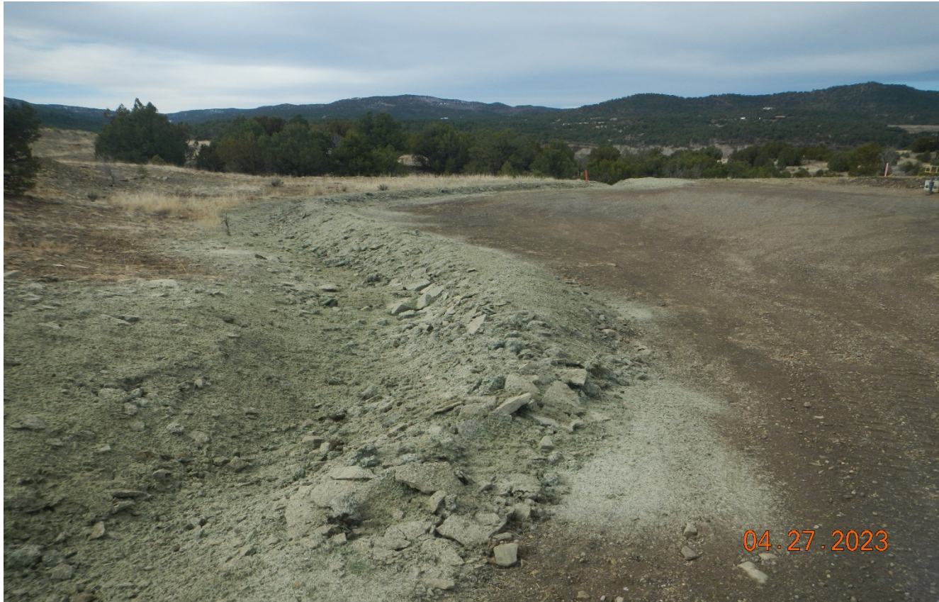
Photo 2. The berm around the east side was repaired and stabilized.
