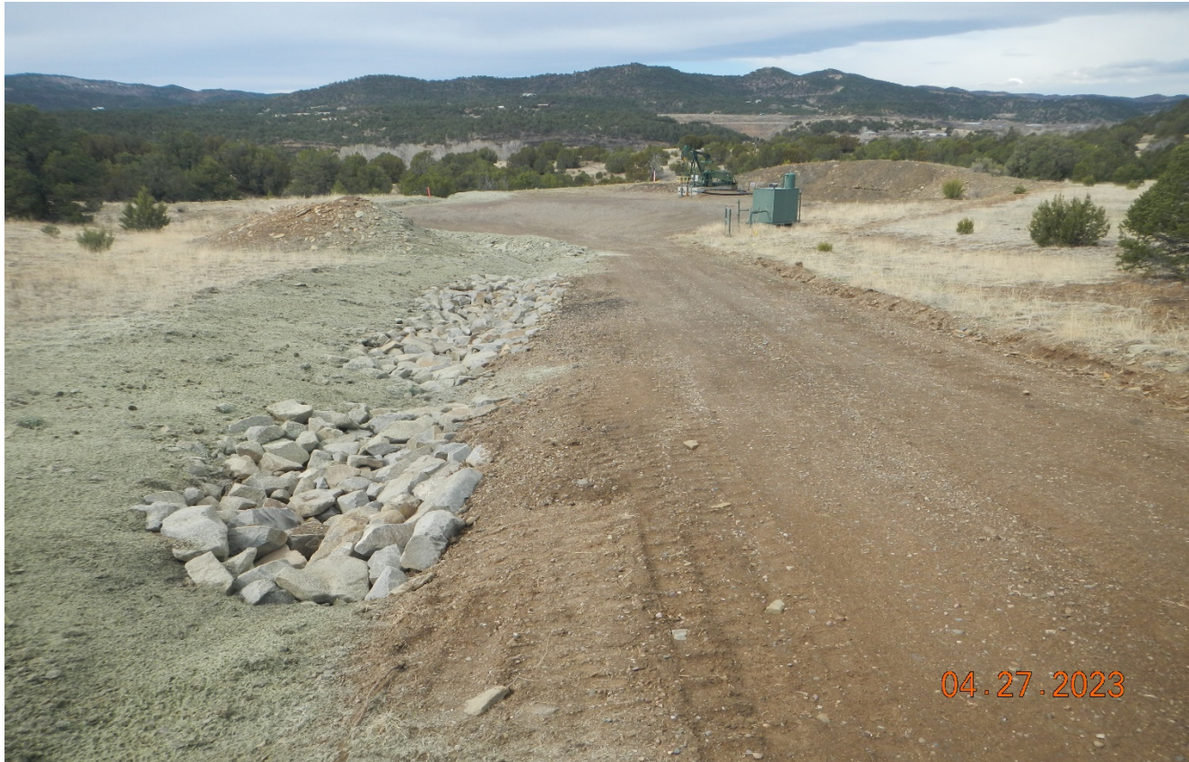
Photo 1. Facing southwest along the access road toward the location. The road side has been repaired and stabilized with rip/rap, seeding, and hydromulch.
