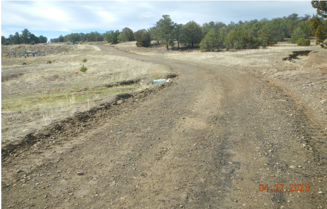
Photo 1. Facing south toward the access road. The erosion along the road and culvert outlet was repaired.
