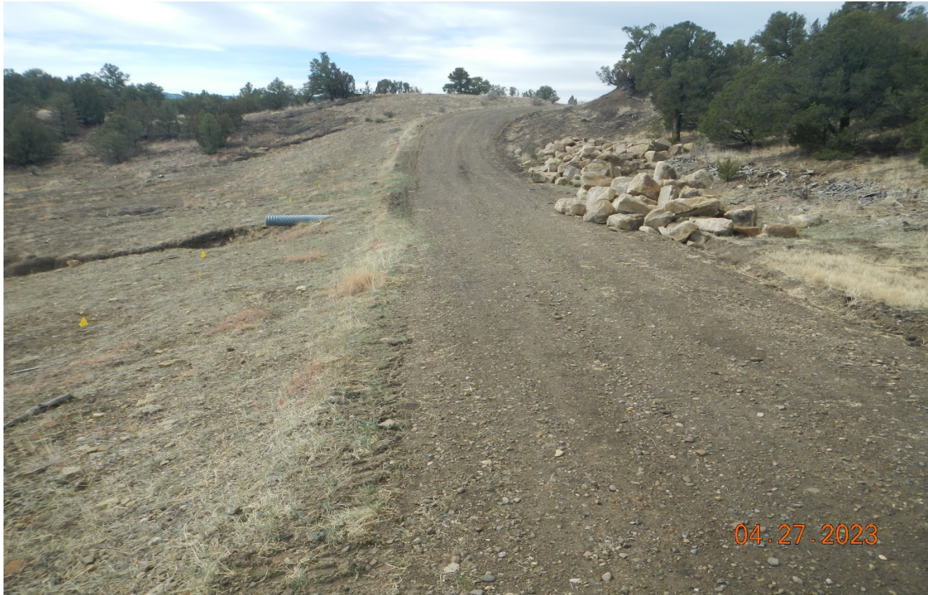
Photo 3. Along the main road at Lat/Long:37.14002,-104.68079. There is rock rip/rap that has been hauled into this area for repair of the culvert outlet erosion.
