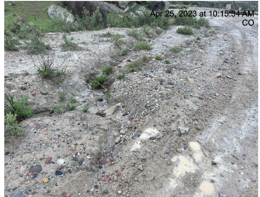
Photo # 6276 Erosion on edge of spur road near ditch
