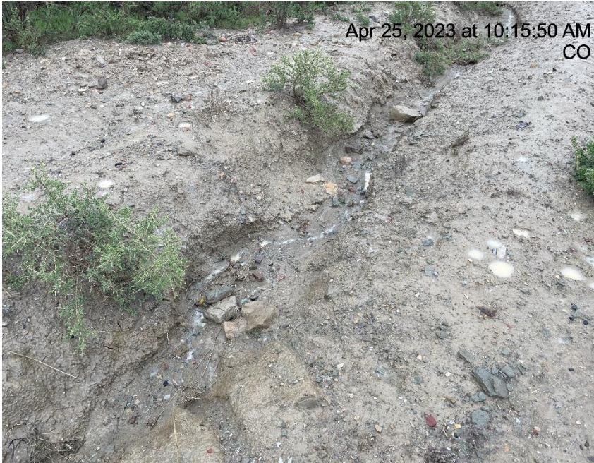
Photo # 6277 Check dam needs maintenance (in ditch along spur road)
