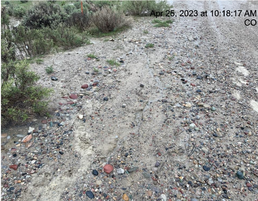
Photo # 6281 Erosion on spur road
