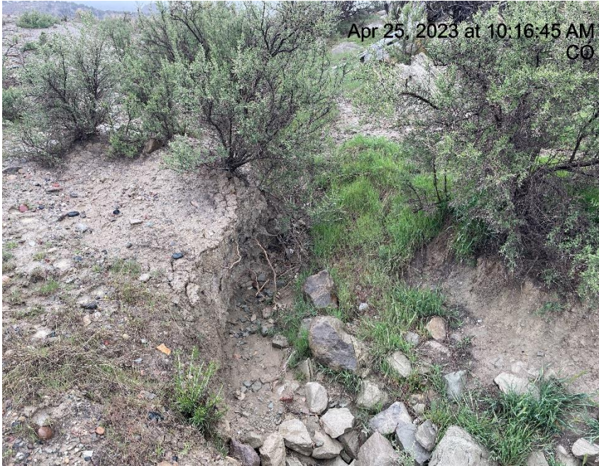
Photo # 6279 Ditch & rip rap need maintenance (along spur road)
