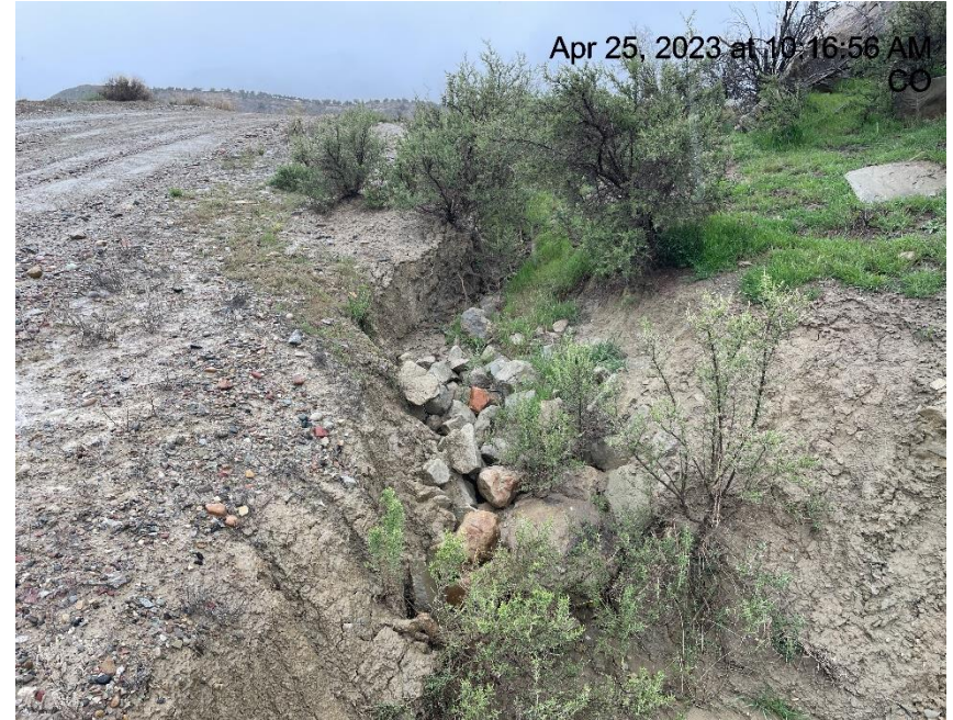
Photo # 6280 Ditch & rip rap need maintenance (along spur road)
