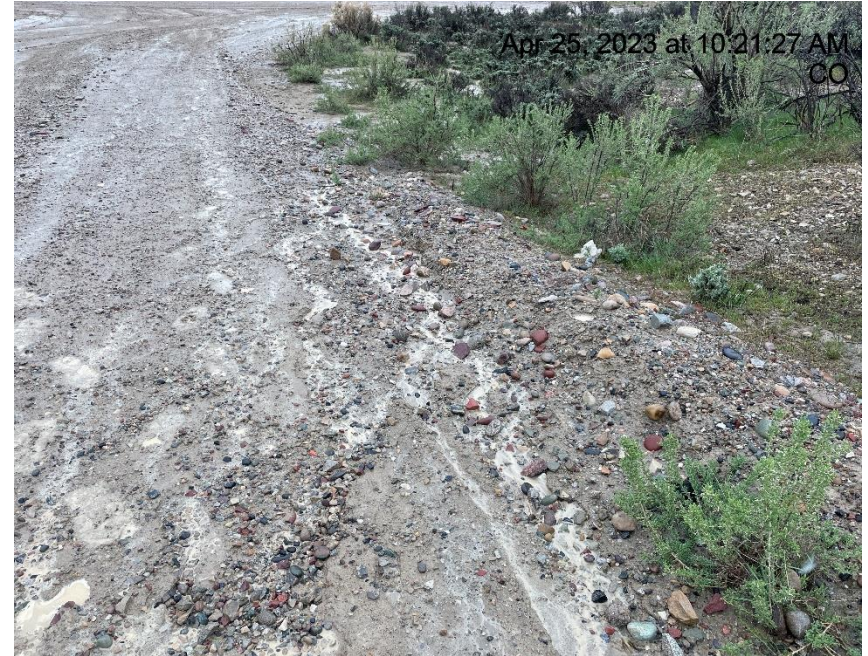
Photo # 6290 Erosion along edge of spur road
