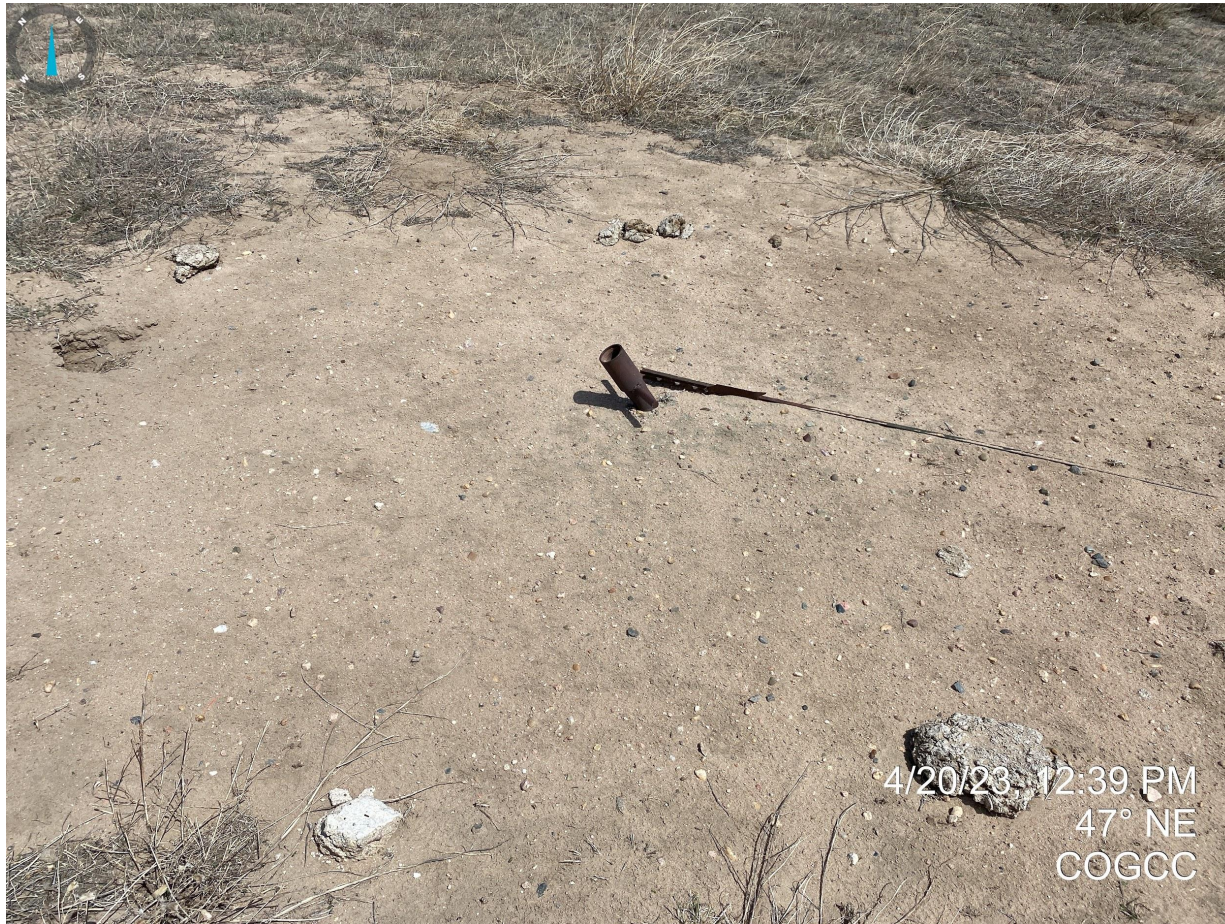
Photo 3. Guyline anchor not properly marked.
