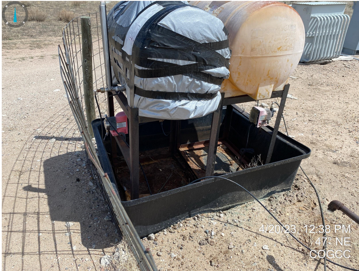
Photo 4. Secondary containment for day tanks at wellhead does not appear to be adequate to contain 150% of the volume of both tanks.
