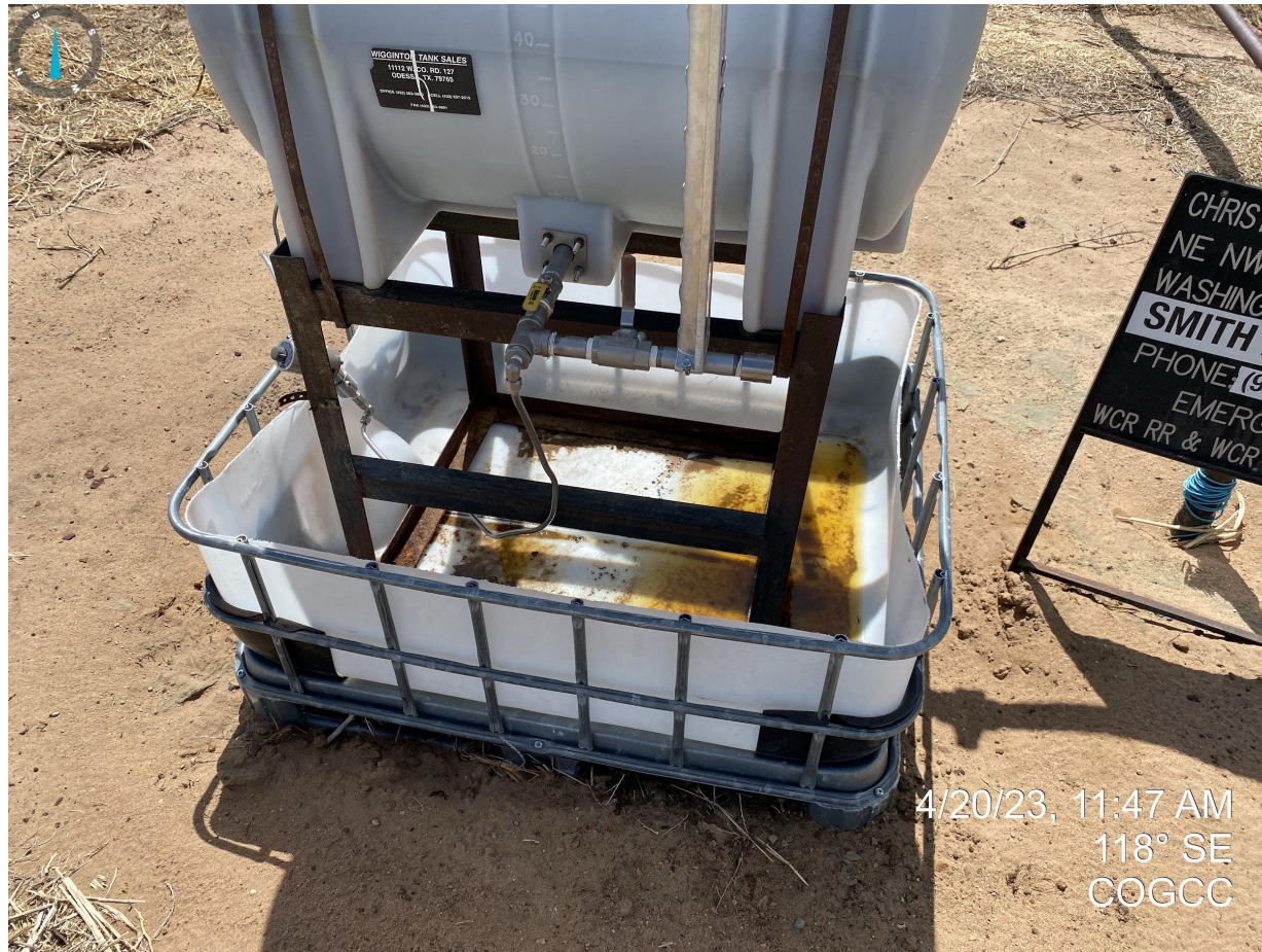
Photo 3. Wildlife netting not installed around secondary containment.
