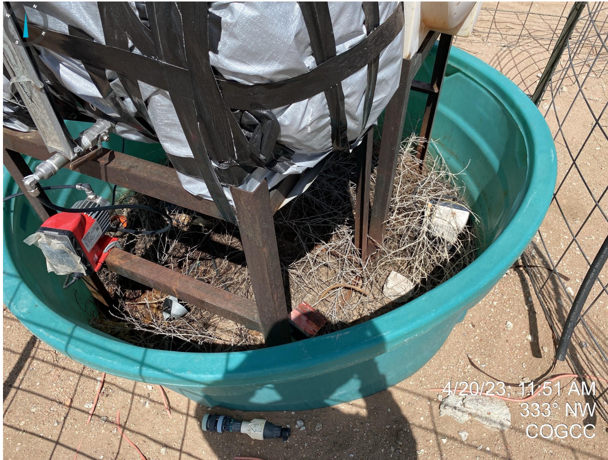
Photo 2. Wildlife netting absent on secondary containment.
