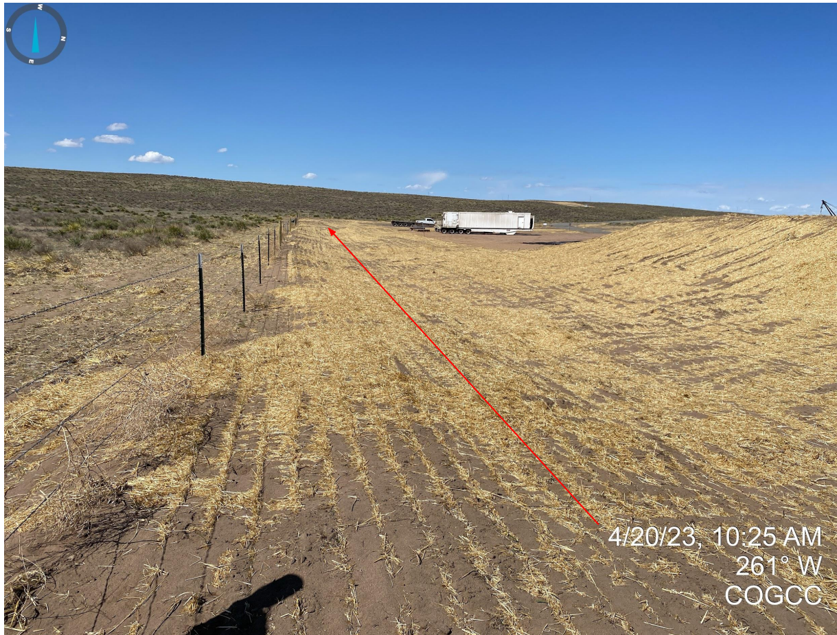
Photo 10. Facing west from the southeastern corner of the location. Topsoil stockpile pictured in the background has been seeded/mulched for long term stabilization. Stormwater BMPs appear to be inadequate along the southern portion of the location.
