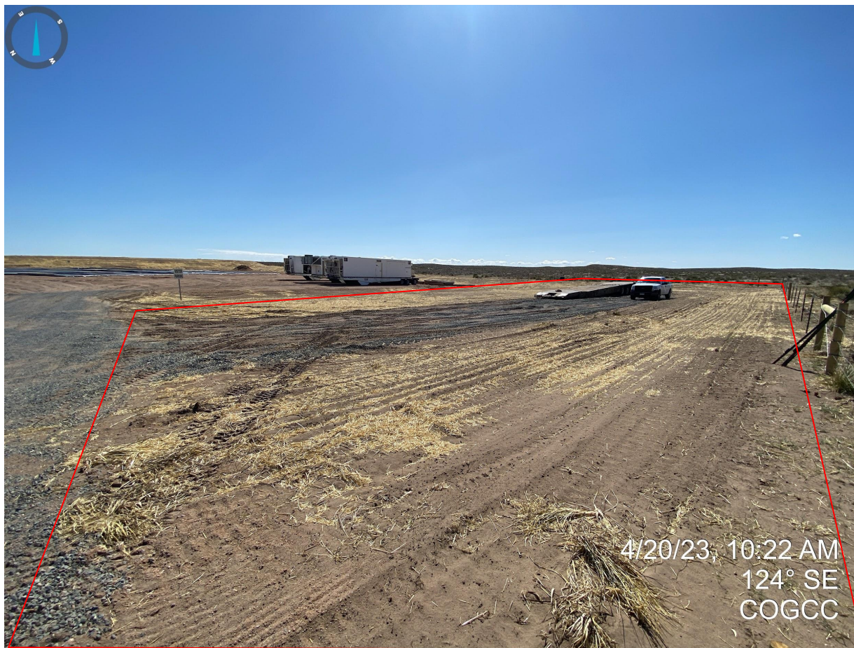
Photo 4. Facing southeast from the location entrance. It does not appear that topsoil have been salvaged from the two “parking areas”; this location is not in compliance with Rule 1002.b. Additionally, no stormwater control BMPs were identified at this portion of the location.
