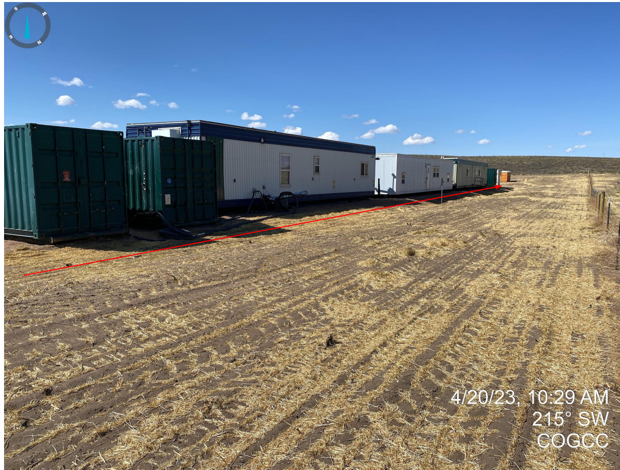
Photo 14. Facing southwest from the northern portion of the location. An interior ditch has been constructed around the production pad and no apparent stormwater BMPs located on the perimeter of the location.
