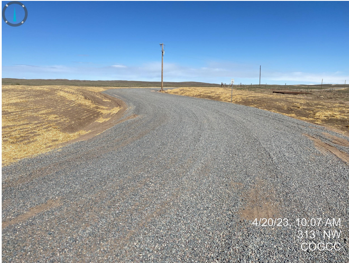
Photo 2. View from access road illustrating that the road has been stabilized with road base and any disturbed areas have been contoured and seeded/mulched for long term stabilization.
