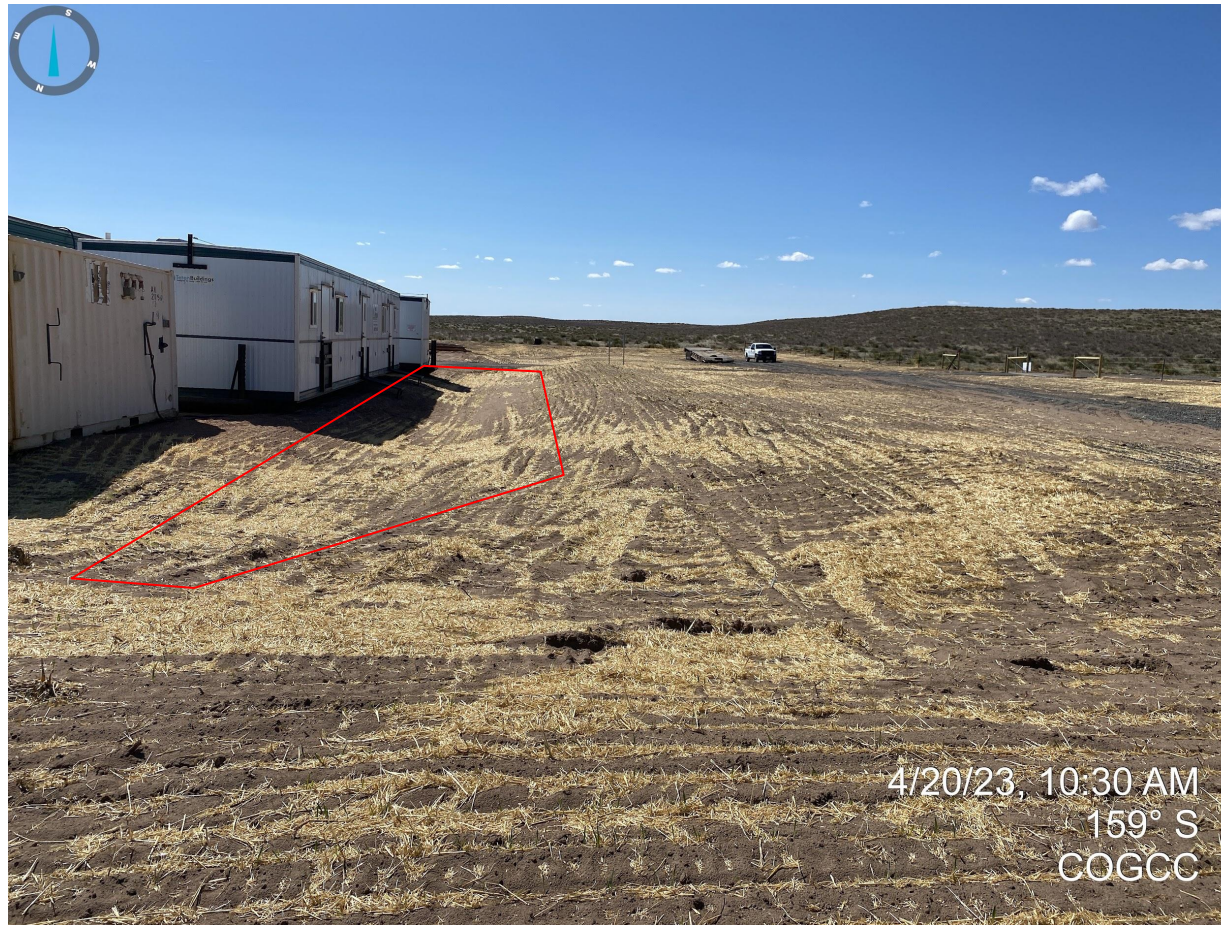
Photo 9. Additional sediment trap installed on the northwest corner of the production area.
