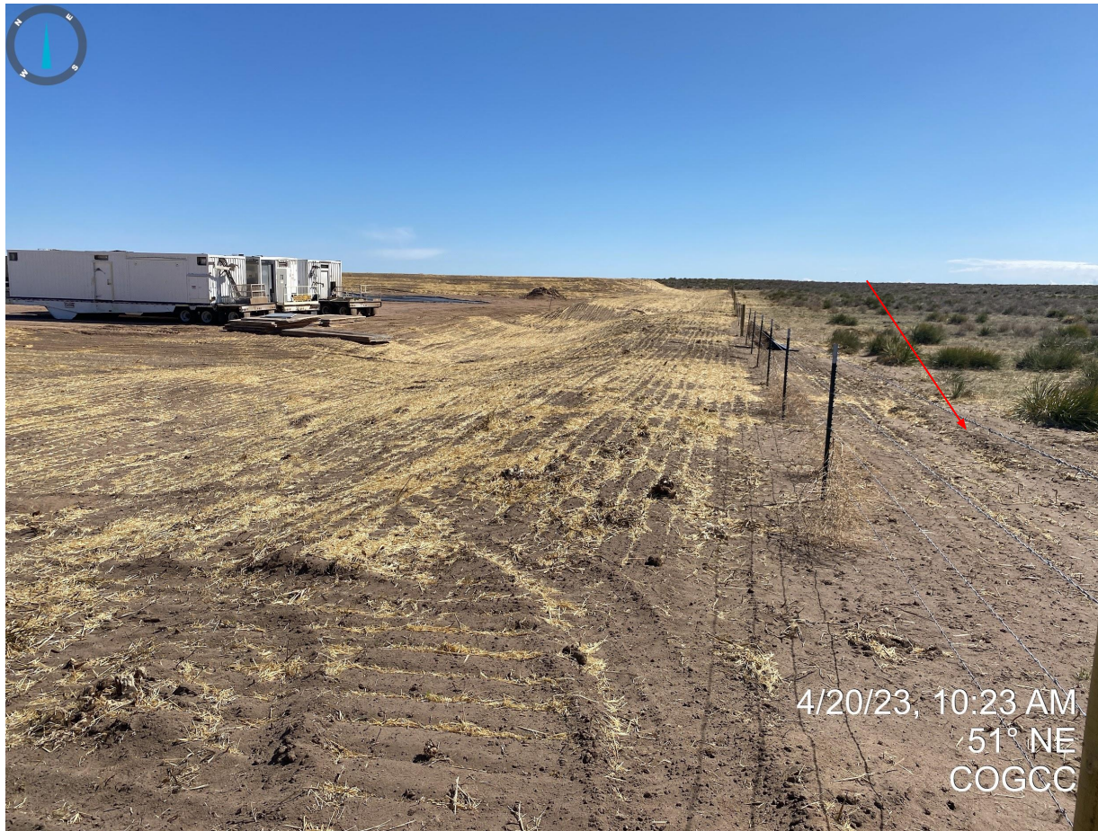
Photo 6. Facing northeast from the southwest corner of the location. Photo illustrates the absence of stormwater control BMPs around the perimeter of the location and additional disturbance outside of the fence line.
