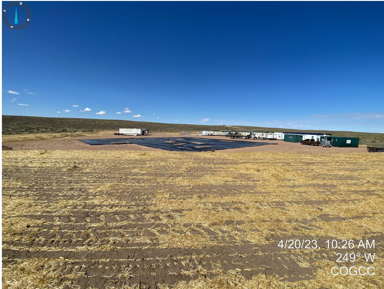
Photo 12. Seeded/mulched topsoil stockpile.
