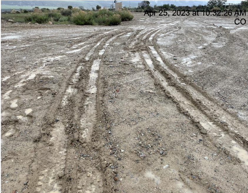
Photo # 6313 Lack of stabilization/compaction
