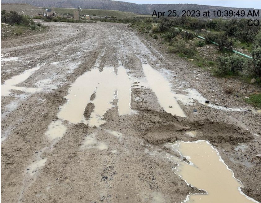
Photo # 6334 Lack of stabilization/compaction
