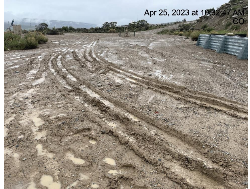
Photo # 6314 Lack of stabilization/compaction
