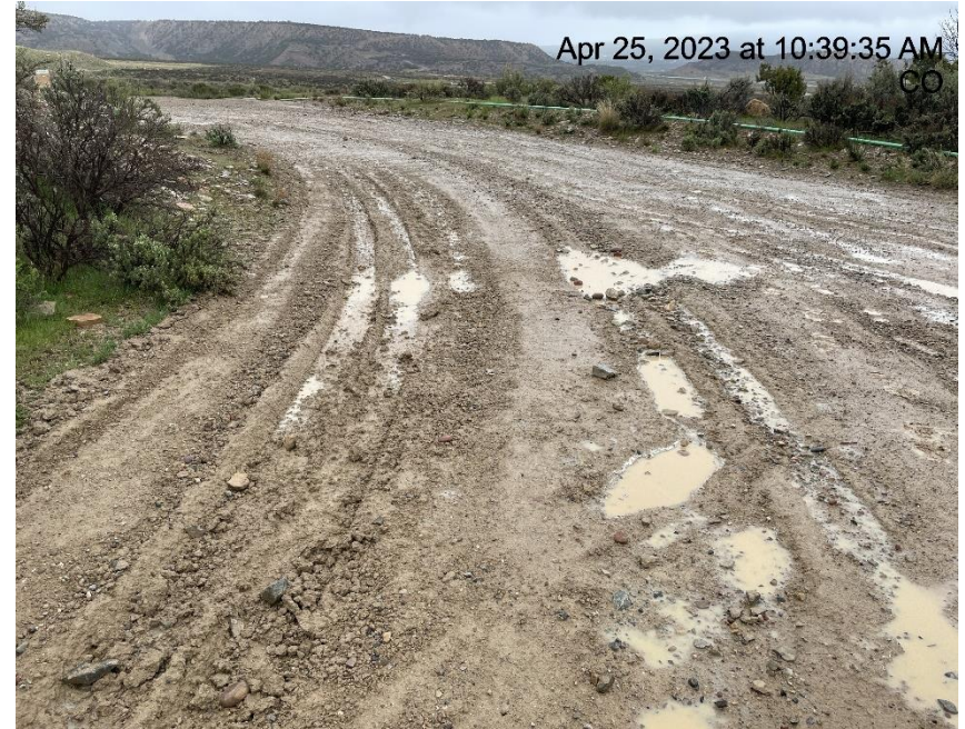
Photo # 6333 Lack of stabilization/compaction
