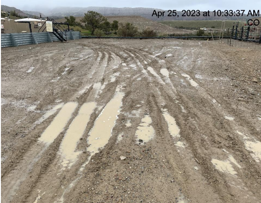
Photo # 6316 Lack of stabilization/compaction
