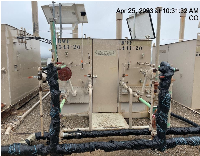
Photo # 6311 Meter calibration info not conspicuously posted
