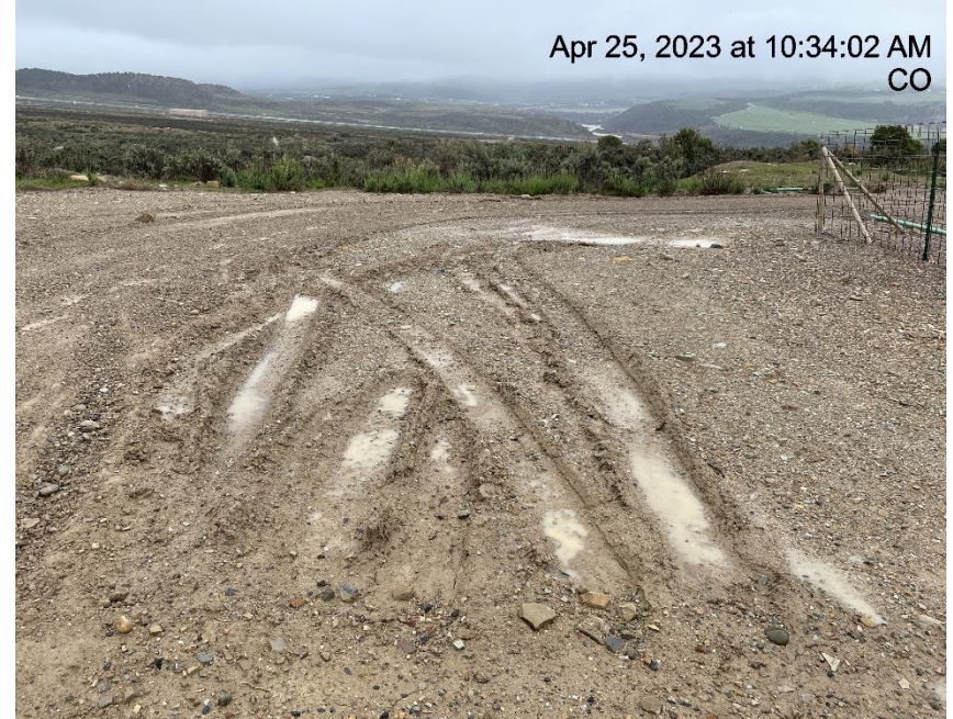
Photo # 6317 Lack of stabilization/compaction
