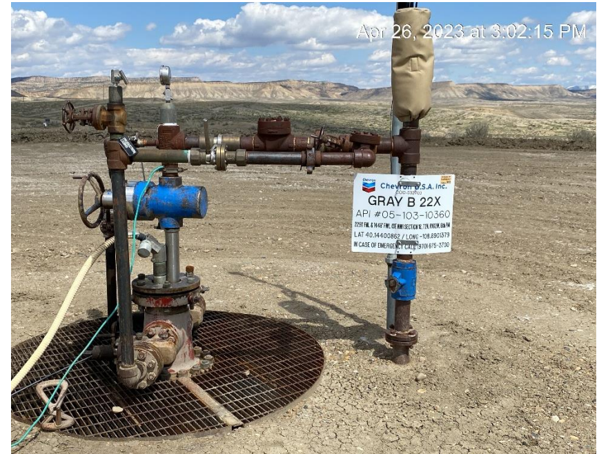
Wellhead and location sign
