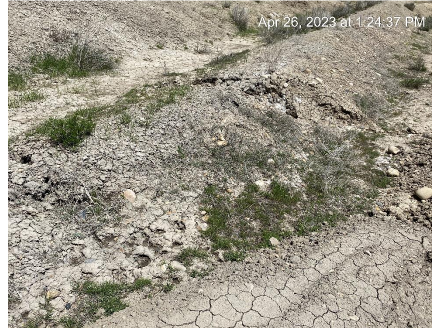
Diversion ditch full of sediment eroding to access road
