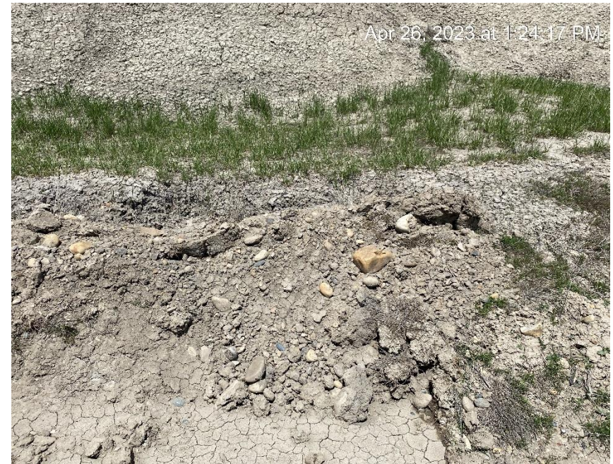
Diversion ditch full of sediment and erosion onto location
