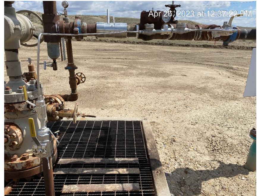
Surface casing hooked into flowline
